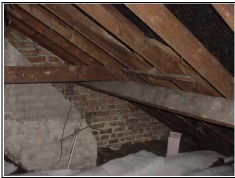
General view of the front roof
