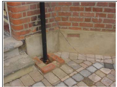
Brick around the gully
