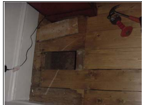
Opening up of the floor to the dining room area
