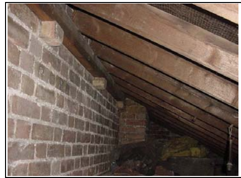
General view of the rear roof
