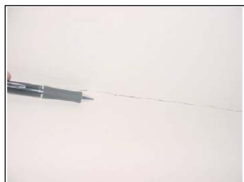
An example of the hairline cracking to the right hand wall of the Kitchen
