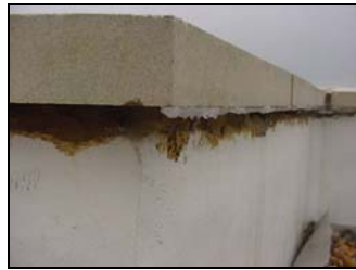
Shows mastic drip has been added
