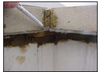
Mastic used to seal joints
