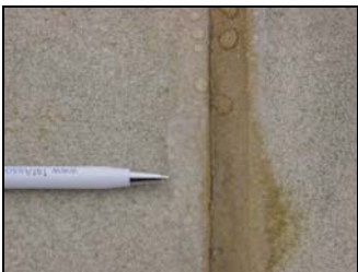
Mastic used to seal joints
