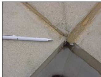
Mastic used to seal joints
