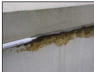
Mastic used to seal joints
