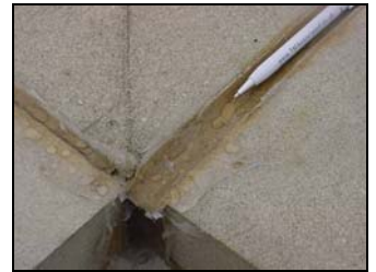
Mastic seal used to seal joints of coping
