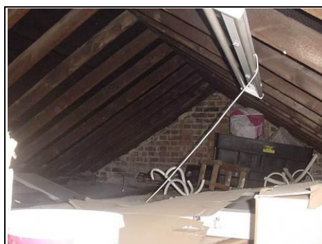
General view of the roof
