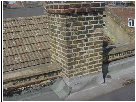
Felt on top of felt around the chimney
