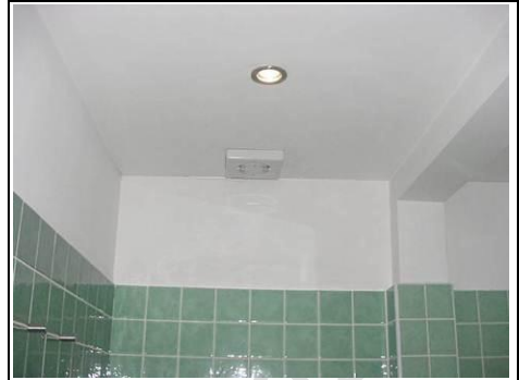
No problems at high level
