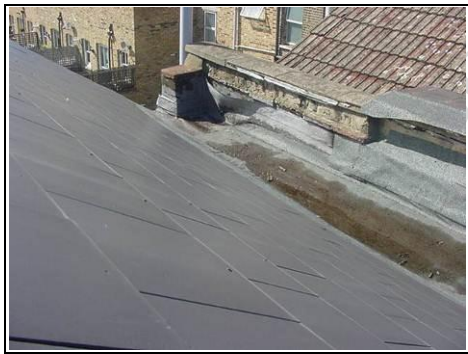
Valley gutter to the right hand side (all directions given as you face the property). This was difficult to view.
