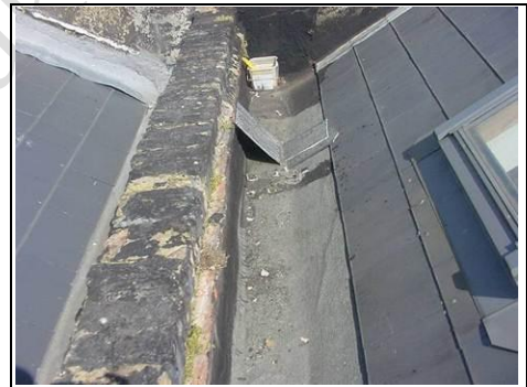
Bitumen paint used
