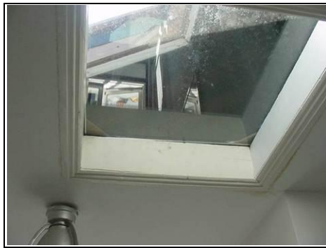
Access onto the roof
