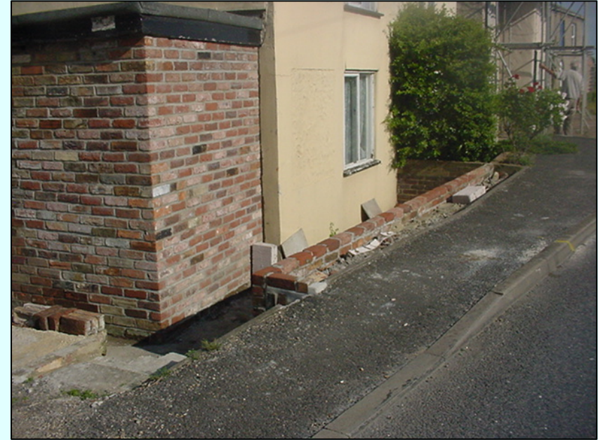
Close up of completed brickwork
