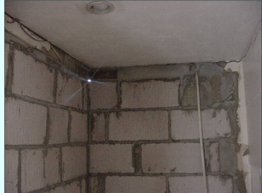
Blockwork up to ceiling height; work progressing on day two.
