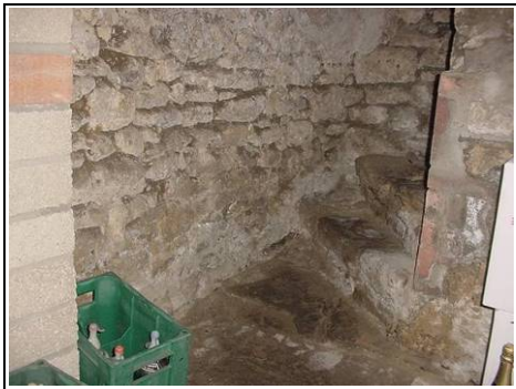
Stairs to Cellar
