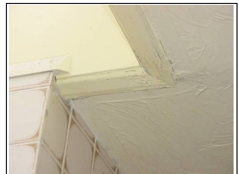
Water leaking through the flat roof.
