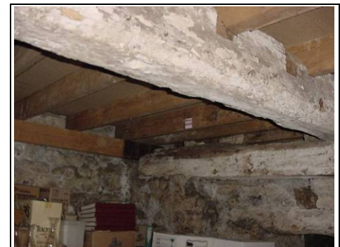
Replaced timbers with central spine beam (white timber)
