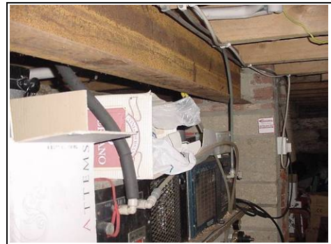
Cellar – note the metal 'I' Beam
