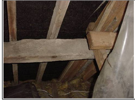
Close up of the purlin
