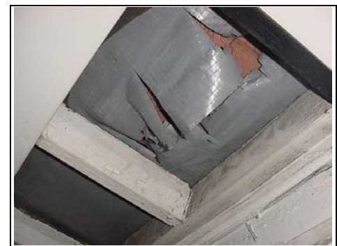
Deteriorating underlayer
