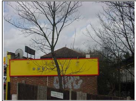
Right hand gable viewed from car park
