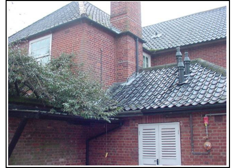
Low level valley gutter
