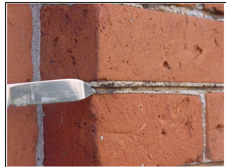
An example of pinch pointing that needs re-pointing
