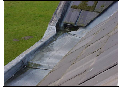
Lead box valley gutter
