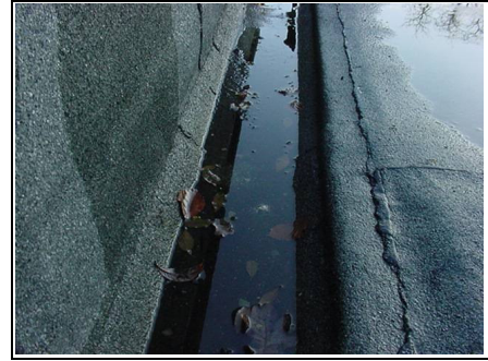
Felt box gutter
