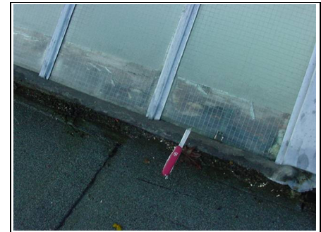
Timber roof light adjacent to flat roofs
