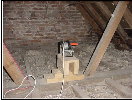
The winch for the chandelier
