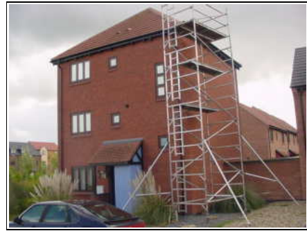
Example of tower scaffold
