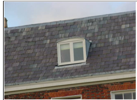
View of front dormer
