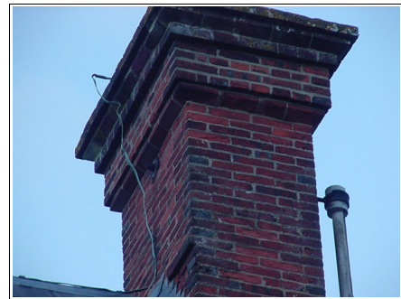
Close up of chimney one
