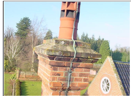
Top of chimney five
