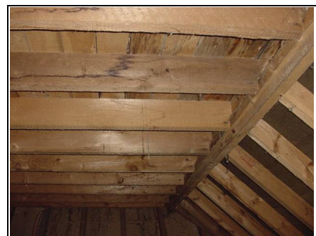
Flat close boarded roof to rear ballroom area
