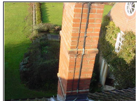
Base of chimney five
