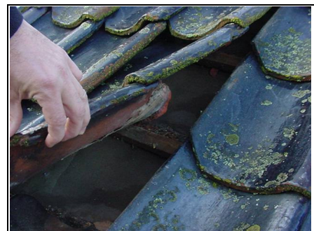
Close up of pantiles
