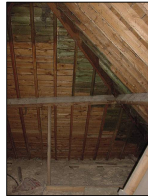
You can see in the purlin that running out in this photo movement has taken place
