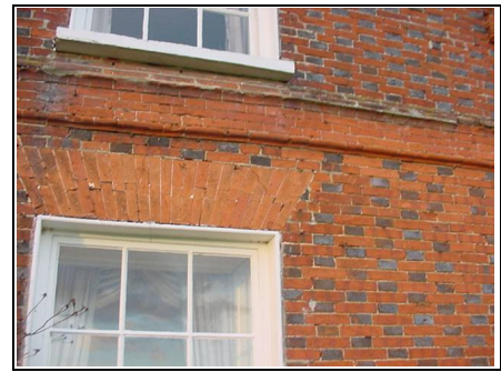
Flemish bond brickwork
