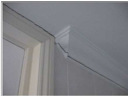
Differential movement in Andrew's Bathroom - further investigation required
