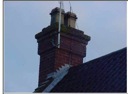
Chimney six – ballroom
