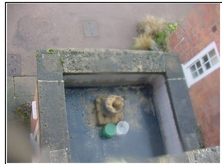
Flat roof over entrance porch
