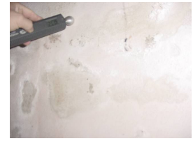
Testing for dampness with Gann Meter
