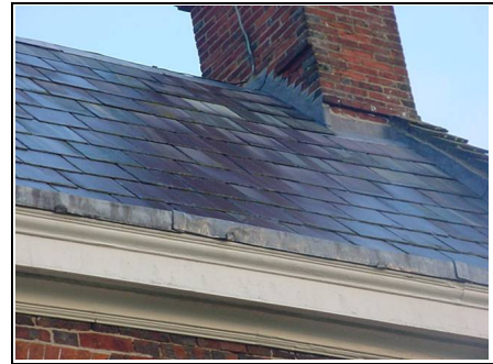
Front south slate roof
