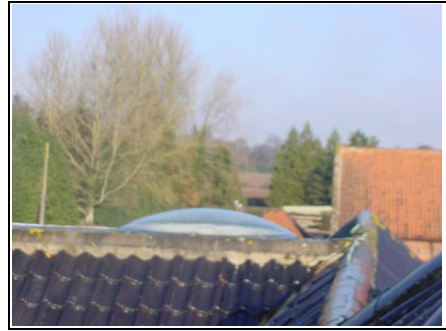
Flat roof over entrance porch
