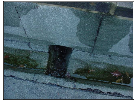
Close up of box valley gutter
