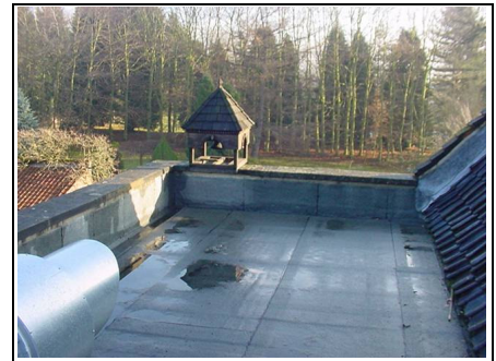
Flat roof near entrance area
