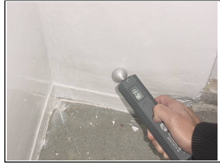
Checking for rising damp
