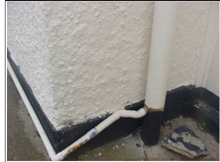
Air vent to left hand side
