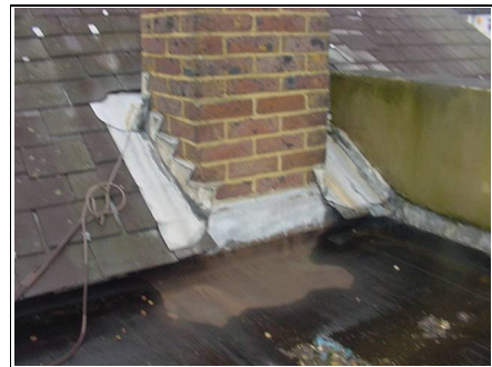
Base of chimney
