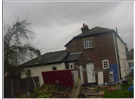
Brickwork rear right hand side, with smooth render to rear left hand side
