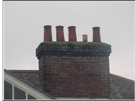
Rear right hand side chimney
