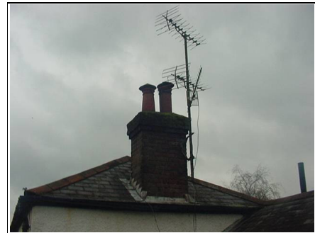
Rear middle chimney
