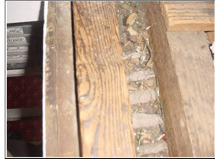
Lath and plaster ceiling
