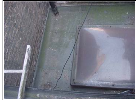
Roof lights have a life of approximately ten years
