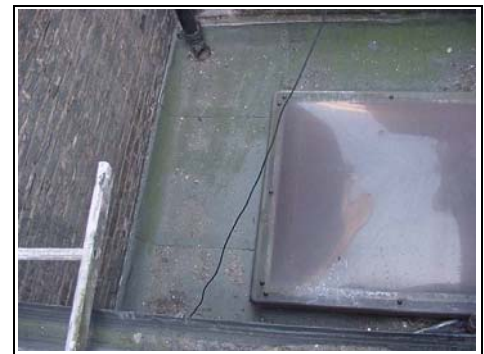
Skylight and discharging downpipe
