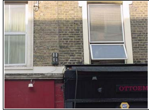
First floor window
