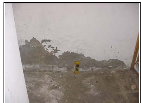
Testing for rising damp
