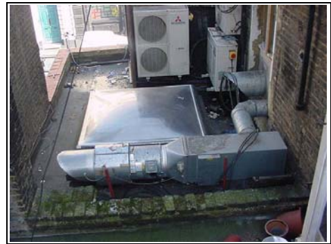
An asphalt covered roof
