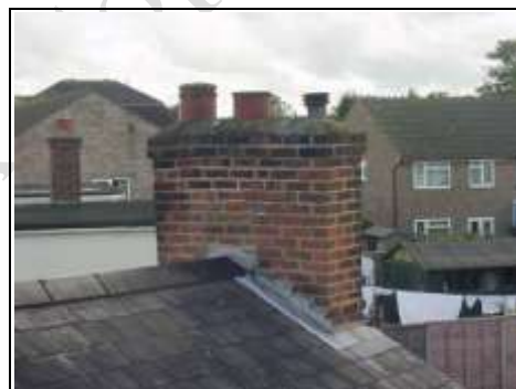
Chimney three located to rear
