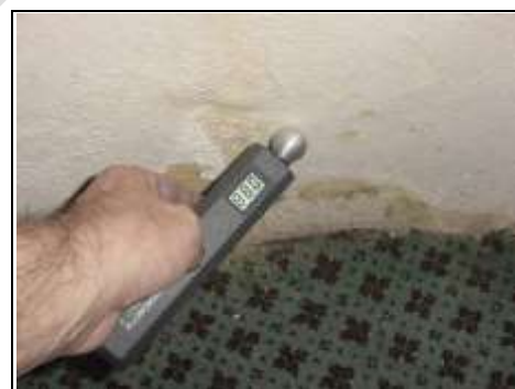
Testing for rising damp in bay window of bar
