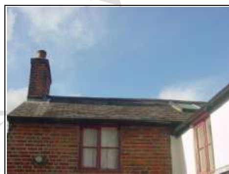
Main roof to rear
