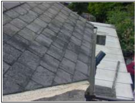
Looking down at the valley gutter
