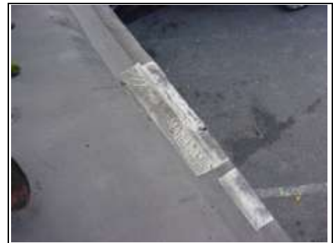
Flashband repair to asphalt roof
