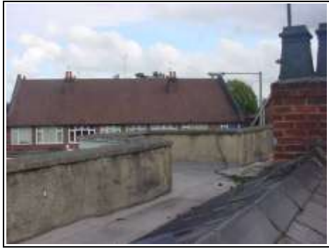
General view of front box gutter
