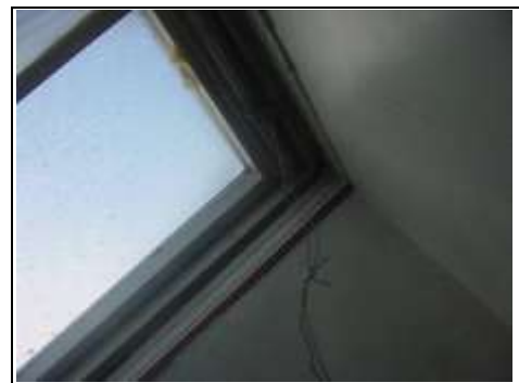
Internal view of roof window
