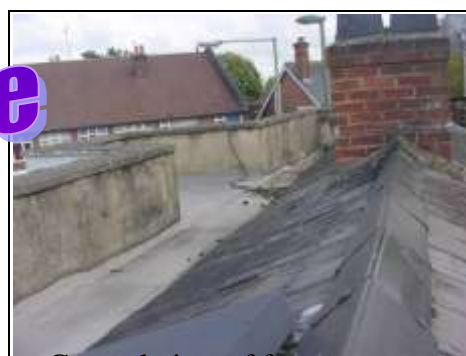
General view of front parapet wall
