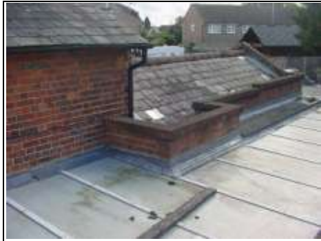
Rear roof parapet wall
