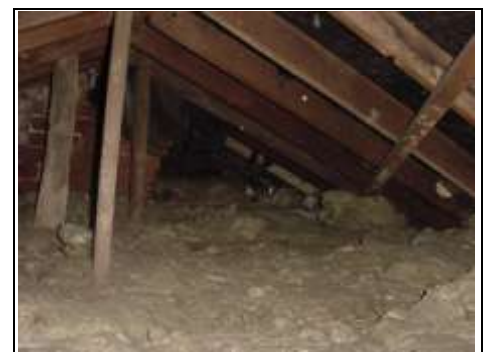
General view of inside of roof
