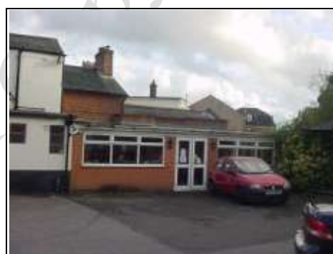
Plastic double glazed windows to conservatory
