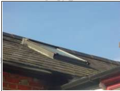
Roof window to rear
