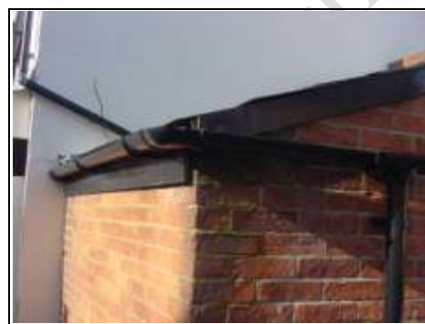
Plastic gutters and downpipes
