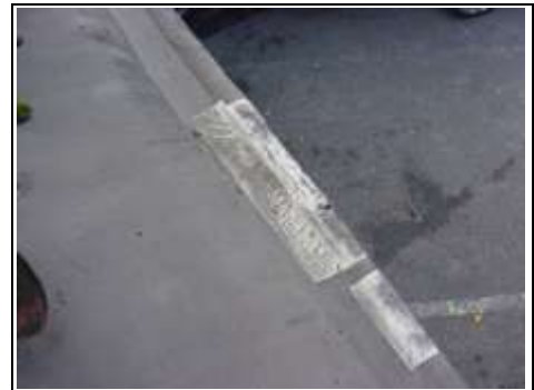
Flashband repair to asphalt roof
