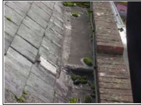
Rear box gutter
