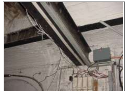
New steels added in basement 12
