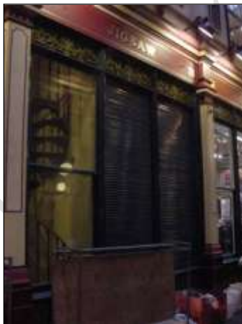
Rear View with access to basement
