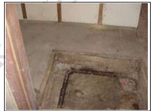
Drain within basement
