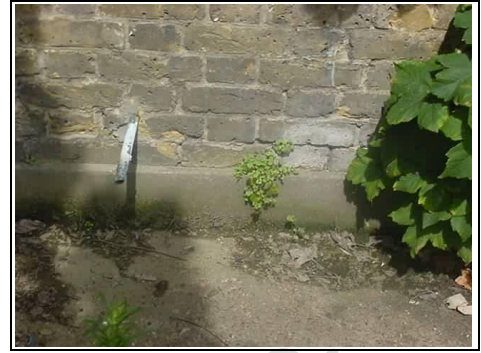
Plants growing within the wall indicate dampness
