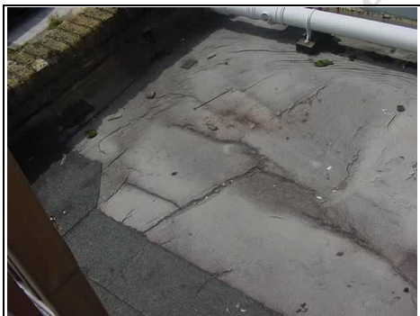
Asphalt felt roof has been repaired
