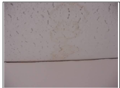
Dampness coming through to ceiling tiles
