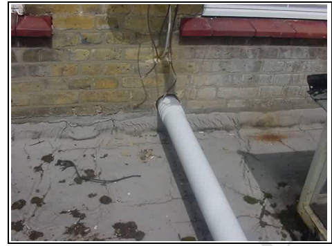
No flashing around soil and vent pipes
