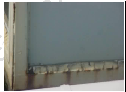
The window frame is starting to rust
