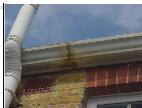
Ogee cast iron gutter is rusting
