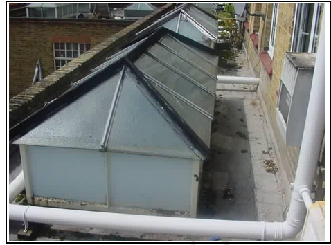
Old style roof window on flat asphalt roof
