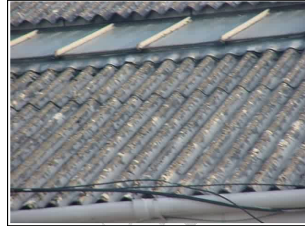
Asbestos roof
