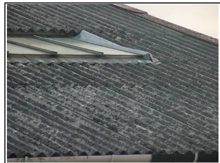
Asbestos roof on Unit X and Y
