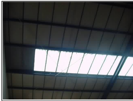
GWPP roof light
