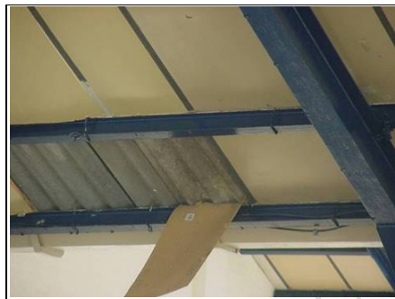
Under cladding coming down
