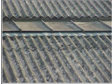
Asbestos roof
