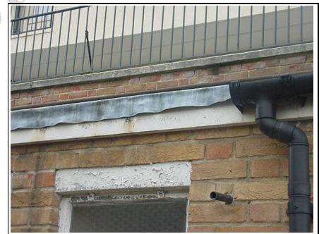
Missing gutter
