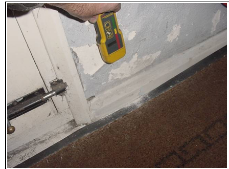
Testing for rising damp
