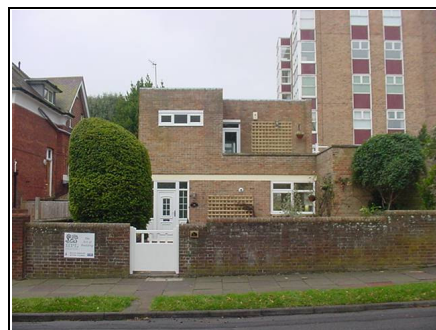
1960's concrete frame
