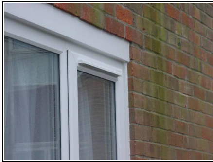
Concrete lintel visible externally but they are not always visible
