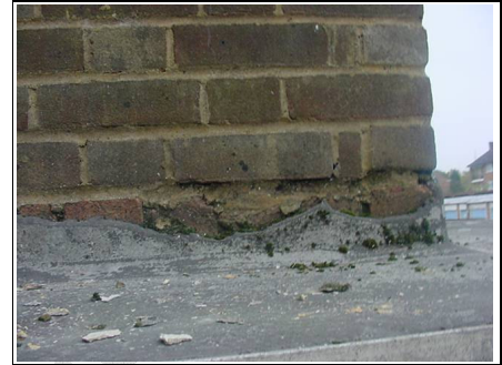
Damaged flashing
