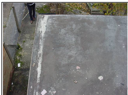
Rear flat roof over toilet area
