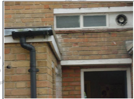
Missing gutter
