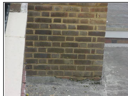
Damaged flashing
