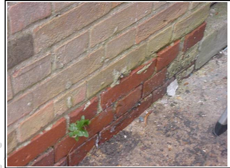
Brickwork to base of property
