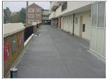
Walkway/balcony to rear of property
