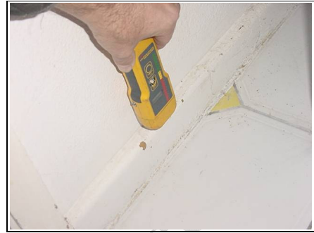
Testing for rising damp
