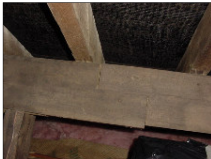
Close up of one of the purlins.
