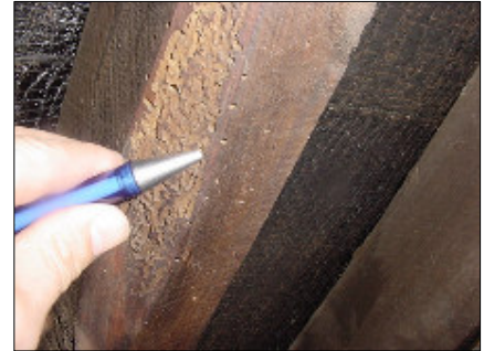
The worst area of woodworm that we could find.
