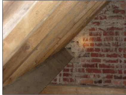
Another general view of the roof.
