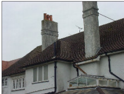
The two rear chimneys.
