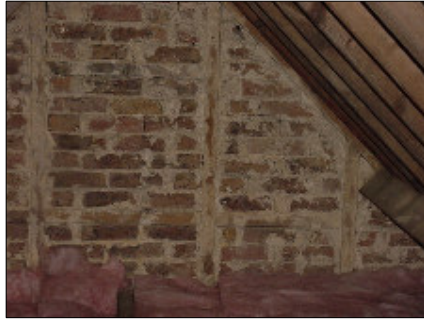
Close up of the timbers in the walls.
