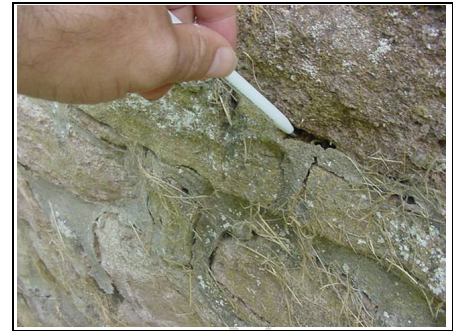
Wall with cement mortar
