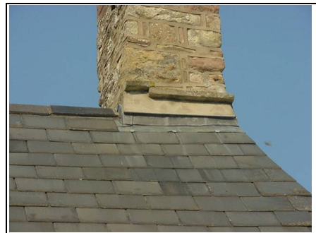
Base of Chimney one
