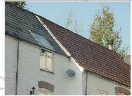
Slate and tile roof meet
