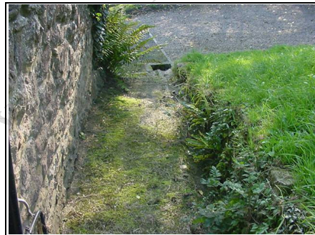
Gulley to the drain
