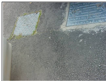
Manhole we didn't open
