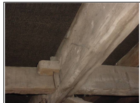
Peg fixing within right hand side roof
