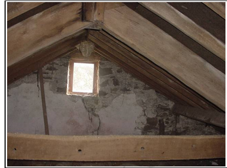
Roof over bedrooms right hand side
