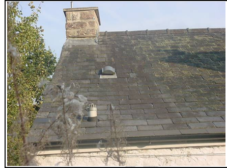
Vent in roof
