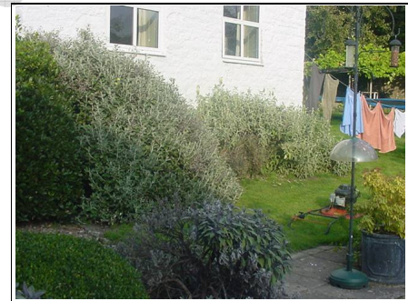
Plants growing around base of property
