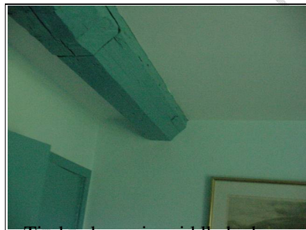
Timber beam in middle bedroom right hand side
