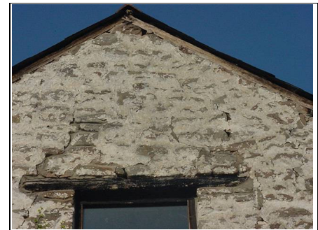
Timber lintel to barn
