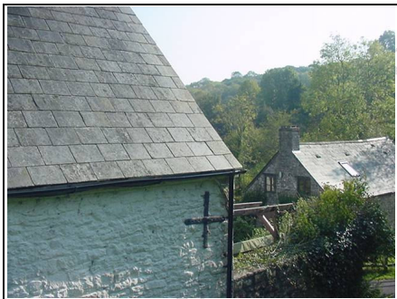
Slate roof left hand side front
