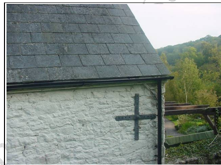
Tie in wall
