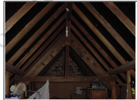
Roof over kitchen
