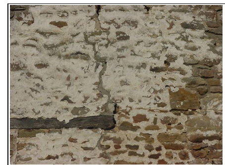
Barn – where you can see bearing or bonding timbers
