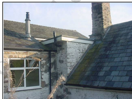
Close up of flat roof
