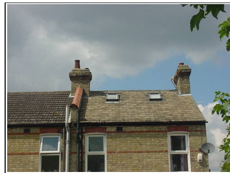
Main roof from rear
