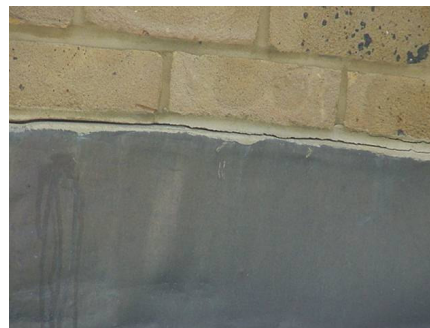
Hairline cracking
