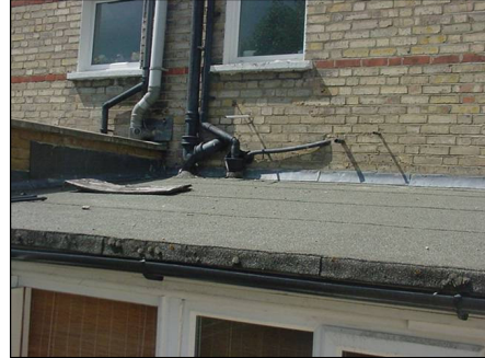
Flat roof to rear of property
