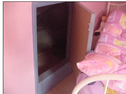
Access to the roof
