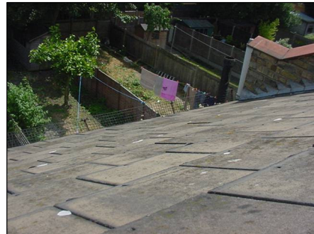
Asbestos slates
