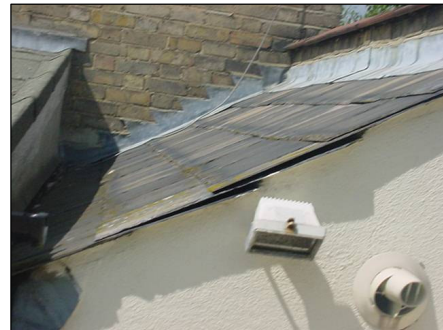
Valley gutter to the pitched roof
