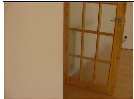
Glass door without any safety glass
