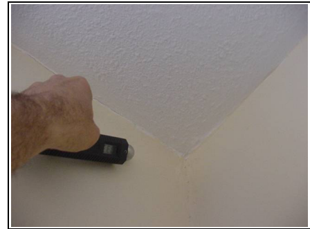
Checking for lateral dampness but property dry lined
