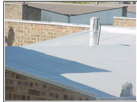
Close up view of roof
