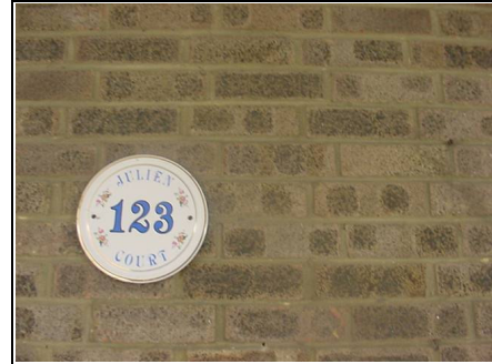
Stretcher Bond brickwork
