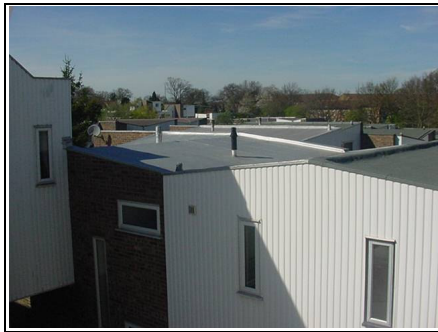
Overview of roof
