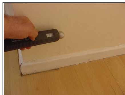
Checking for rising damp
