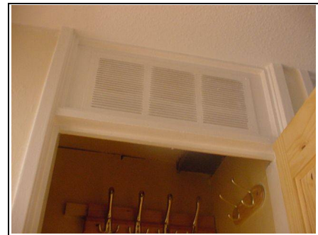
Old air vent for old warm air system
