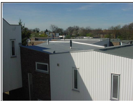
Overview of roof
