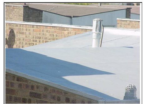
Extreme close up of roof
