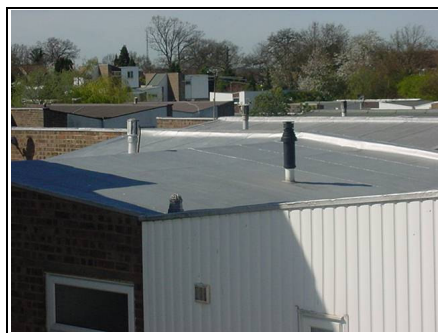
Close up of roof
