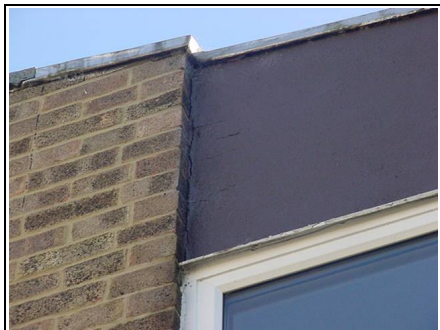
Mastic disintegrating
