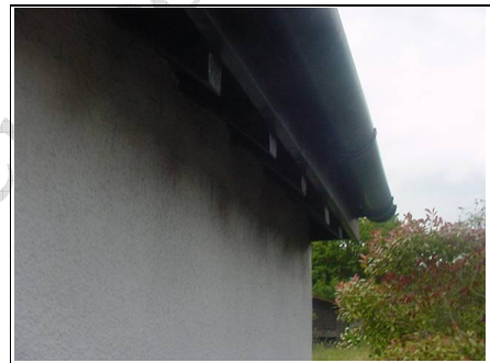
Exposed rafter feet
