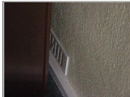
Vent on chimney breast
