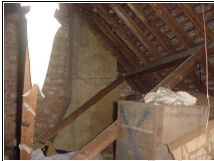
Chimney within roof space
