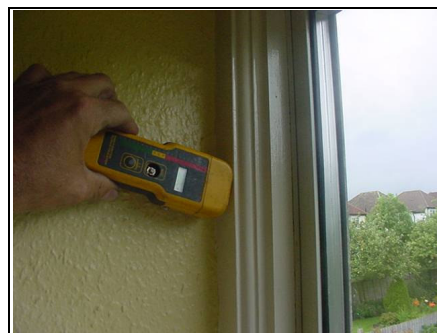
Testing for lateral dampness
