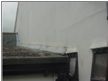
Flashing where garage meets main building
