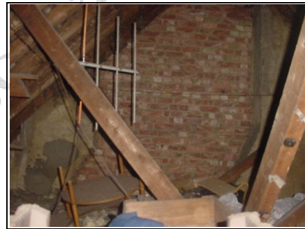
Patch repairs to rendered chimney
