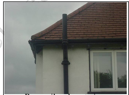
Rear soil and vent pipe
