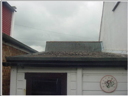
Flat roof to garage
