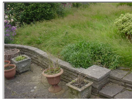
Small retaining wall to rear garden
