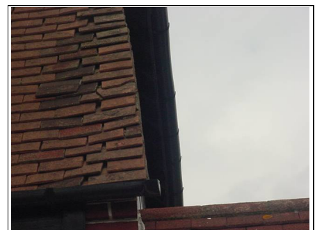
Tiles opened up
