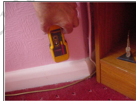
Testing for rising damp
