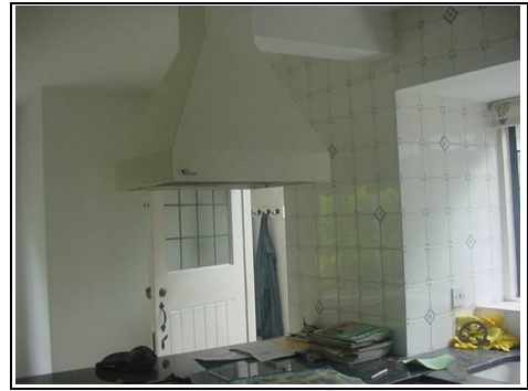
Where the wall has been removed in the kitchen
