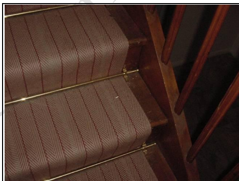
Main staircase ground floor
