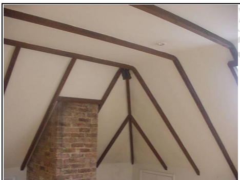
Rooms formed in the roof
