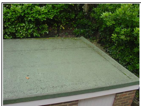
Flat roof on the Garage
