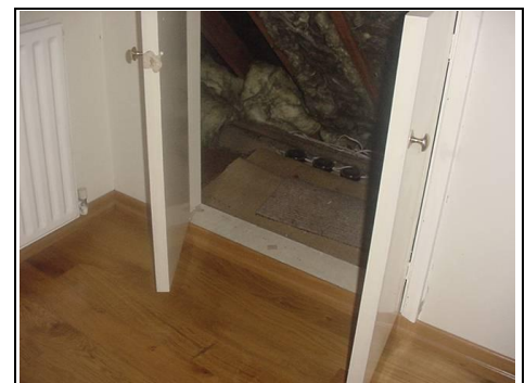
One of the double access doors to enter the roof space
