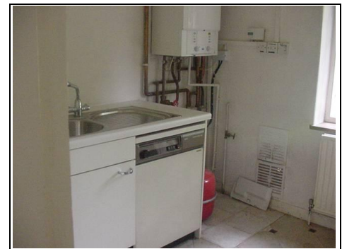
Utility Room (rear left)
