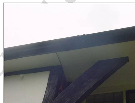
Fascias and soffits
