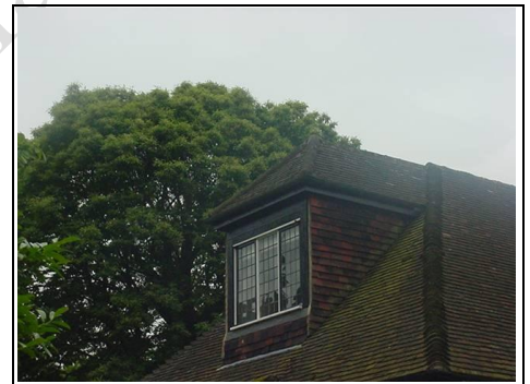
Dormer window left hand side
