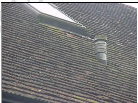
Flue in front roof (left)
