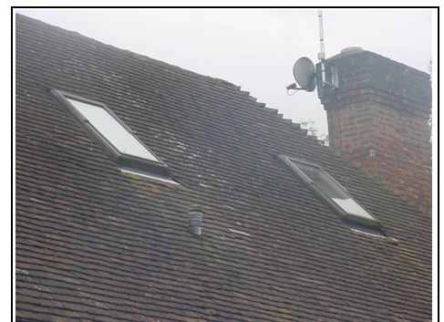
Two roof lights on main roof
