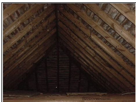
Roof structure over garage
