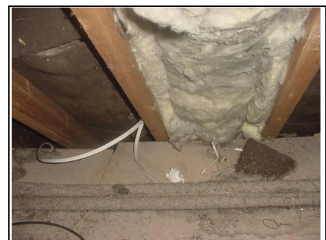
Insulation added in between the common rafters
