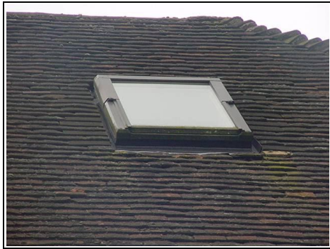
Roof window (right)
