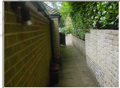
The wall needs weep holes adding to it
