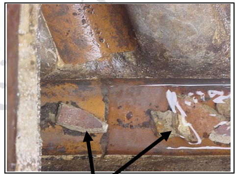
Pieces of pipe visible in the manhole
