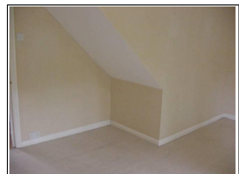
Lined underside of the stairs- middle rear bedroom – first floor
