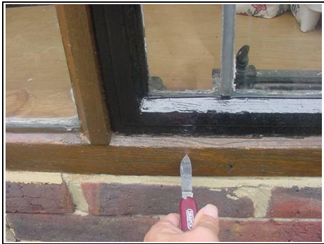
Knife testing window to the rear right of the property
