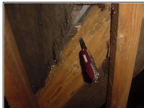
Testing the timber to the front of the property
