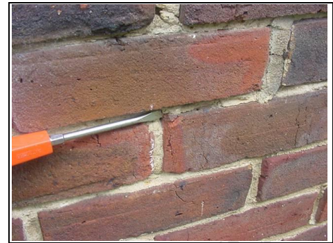
Re-pointing is necessary
