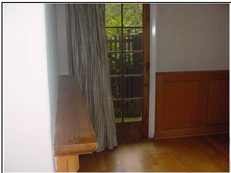
Glazed doors may be a security risk
