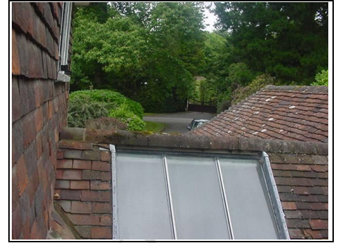
Roof window left entrance
