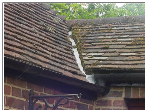
Pitched roof where it meets the walkthrough roof
