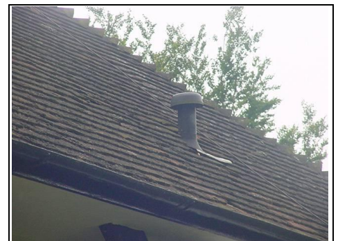
Flue in front roof (right)
