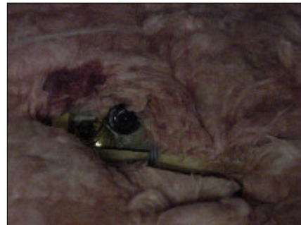
The insulation starting to cover the ceiling lights.
