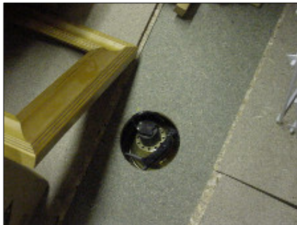
Ceiling light cut around.
