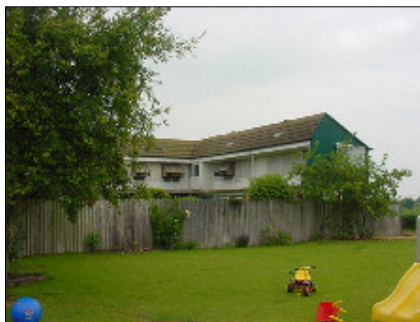
Rear Elevation With next door's huge Pigeon Loft
