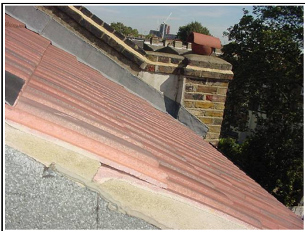
Close up of roof tiles
