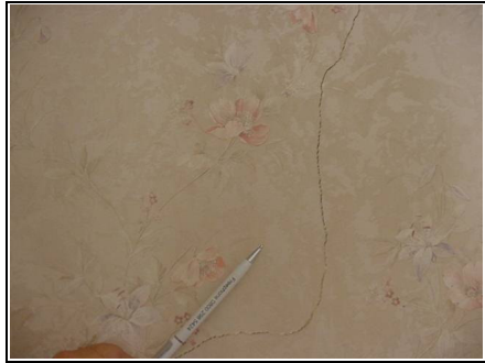
Vertical cracking
