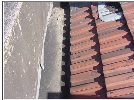
Close up of box valley gutter.
