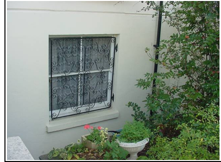
Movement can be seen on the walls
