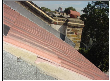
Close up of concrete roof tiles
