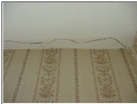
Cracked ceiling
