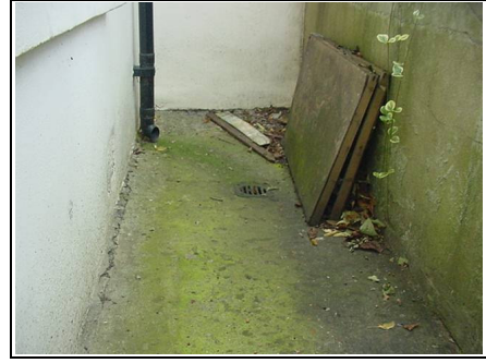
A photo of the downpipe discharging to the base
