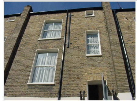
Flemish Bond brickwork to the rear
