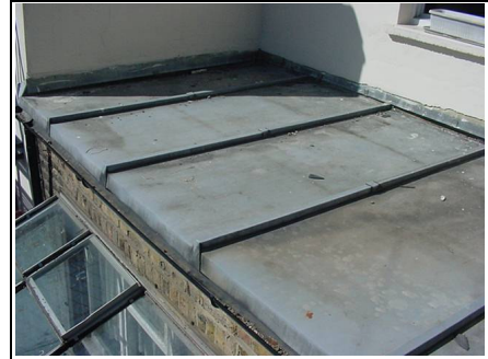
Downstairs flat roof; metal covered
