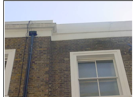
Rainwater downpipes and hopper head
