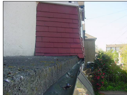
Front flat roof
