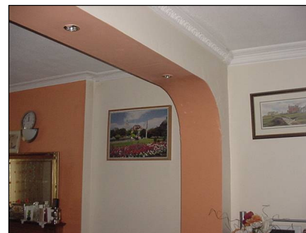
Removal of wall
