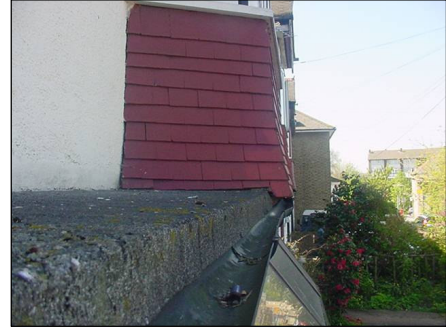
Poor quality front flat roof
