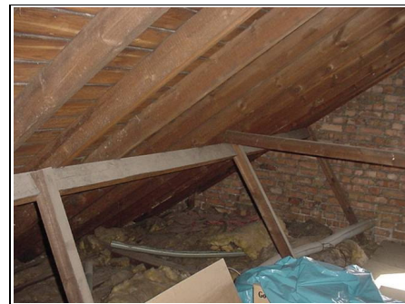
Cut timber roof with close boarding
