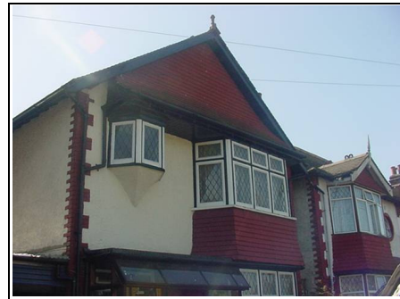
General view of main roof
