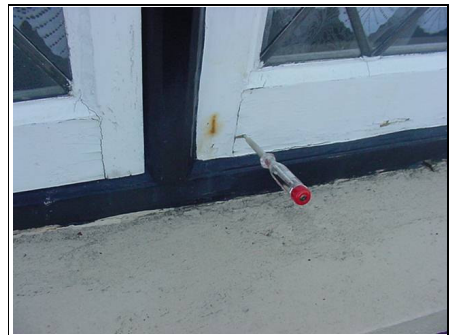
Timber degrading
