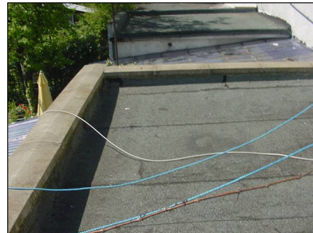
Rear flat roof
