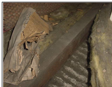
Lath and plaster ceiling
