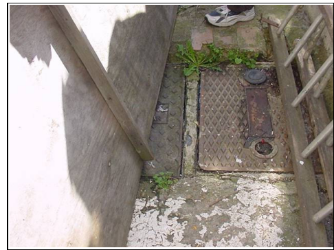
Drain at rear right hand side on next door neighbour's land
