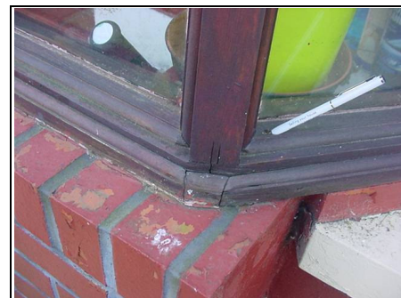
Testing for wet rot at front window
