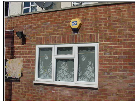
Stretcher bond brickwork to rear extension
