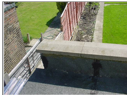
Parapet wall to flat roof
