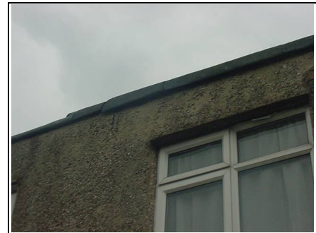
Pebbledash starting to deteriorate
