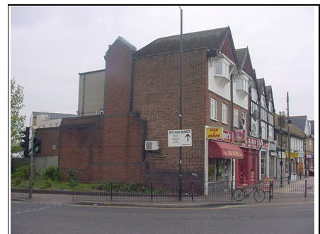
Low level first floor flat roof
