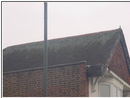
Box gutter on left hand side
