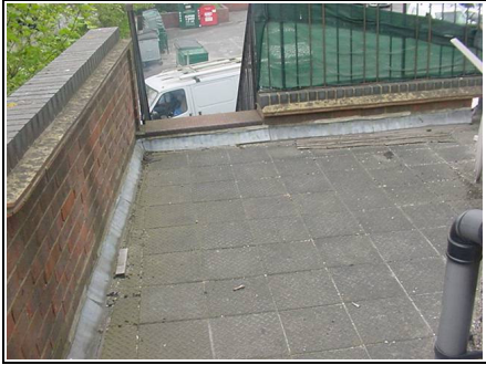
Low level first floor flat roof
