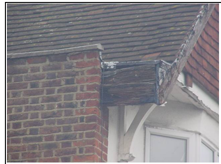
Close up of box gutter
