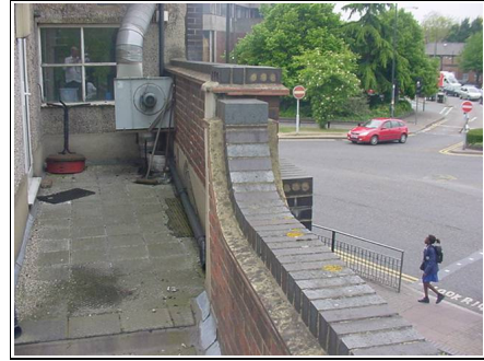
Brick coping and tile on edge
