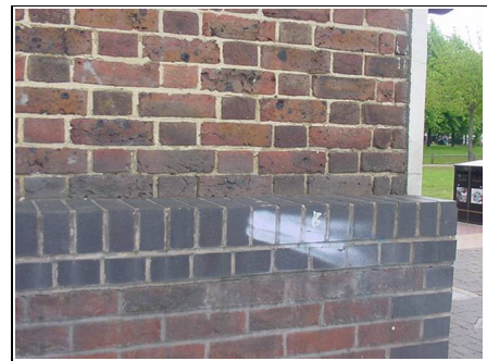
Flemish Bond brickwork
