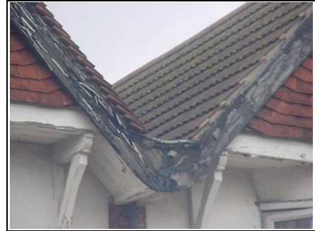
Leaking valley gutter on right hand side
