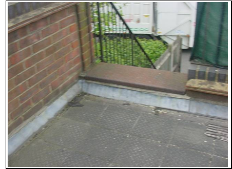
Low level first floor flat roof
