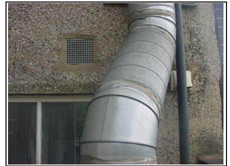
Taping of the joints to the flue
