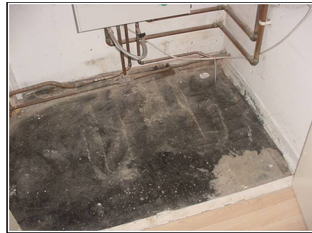
Under the stairs we could see the pitch, which was often applied to the concrete floor finish.
