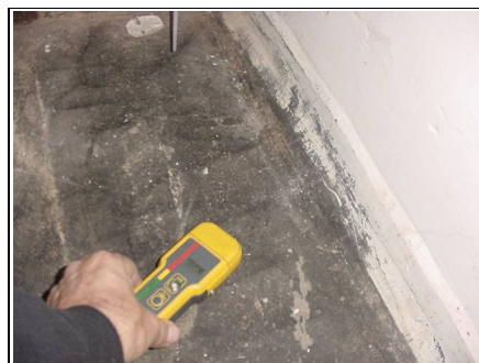
Checking for rising damp
