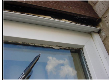
Repair to double glazing on front window
