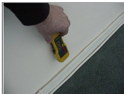
Checking for Rising Damp
