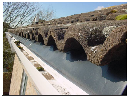
High level guttering
