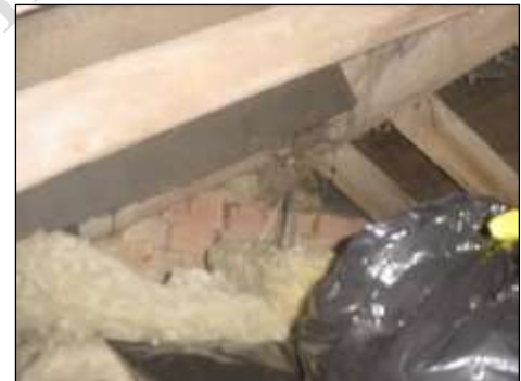
Roof space with a mass of insulation
