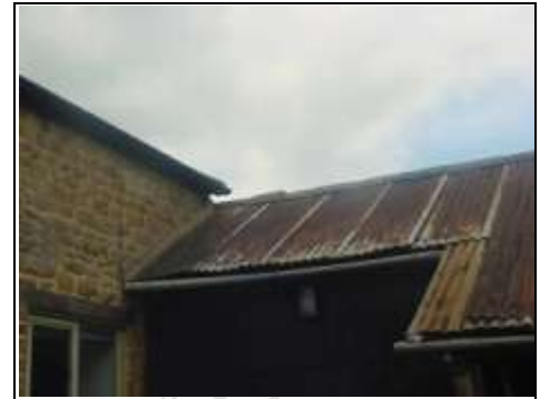
Roof to outbuilding
