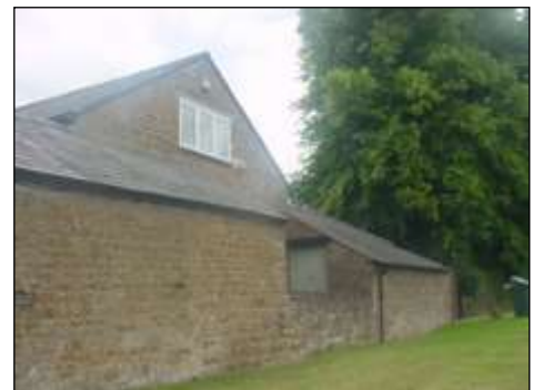
Missing guttering
