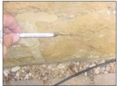
Spalling stonework
