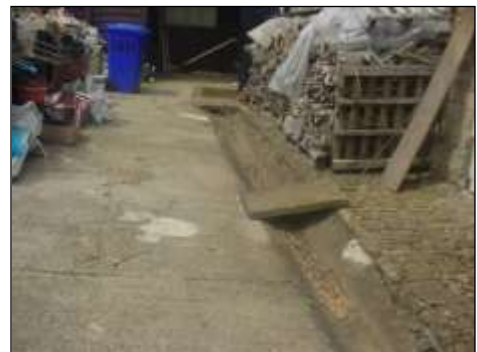
The rainwater gully in the adjoining property
