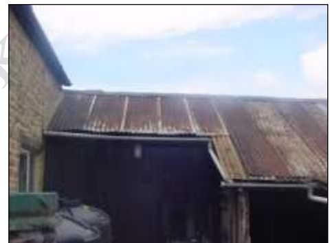
Roof to outbuilding
