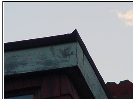
A close up of the fascia and soffit.
