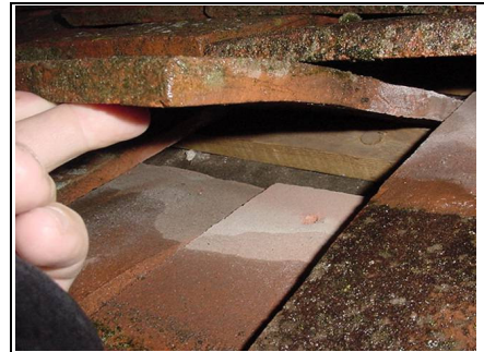
Checking under the tiles
