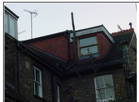
Close-up of rear elevation
