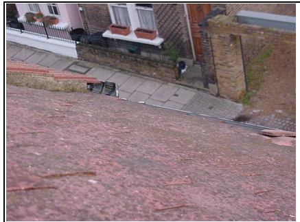
The roof tiles
