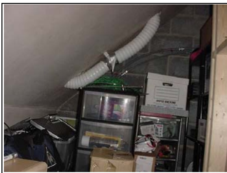
Front Section of Roof
