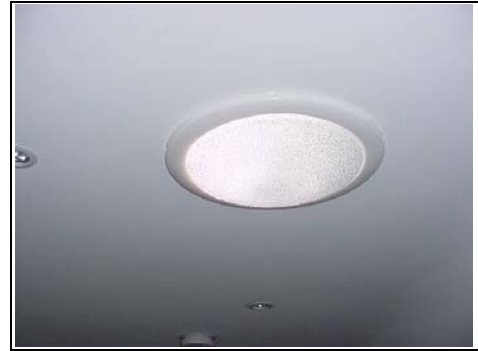
Inside view of the light tunnel
