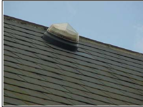
Outside view of the light tunnel
