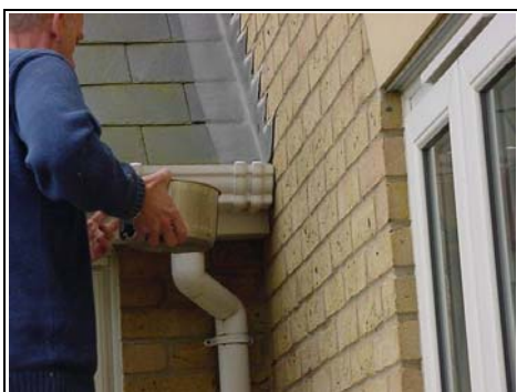
We tipped water down the downpipe
