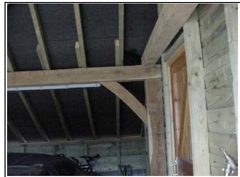
The roof inside the garage
