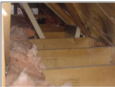
Rear Left Hand Side of Roof
