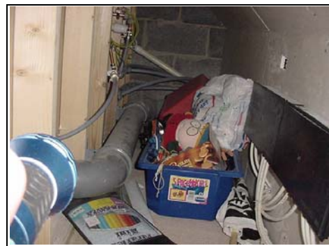
Middle Section of Roof
