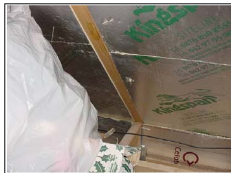
Right Hand Side of Roof
