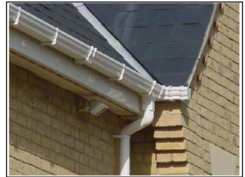
Bottom of the valley gutter where the water can discharge over the gutters during periods of heavy rain fall.
