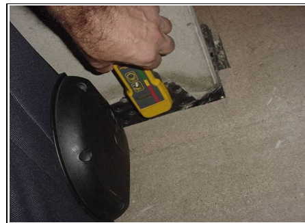
Testing for rising damp
