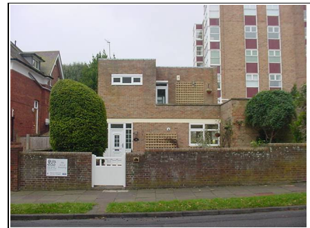
1960's concrete frame
