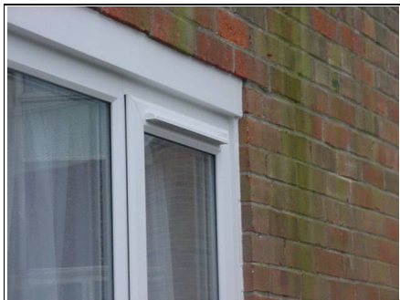
Concrete lintel visible externally but they are not always visible
