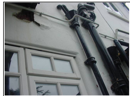
Render deteriorating
