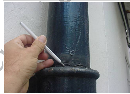
Repairs to soil and vent pipe
