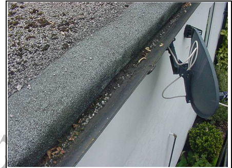
Cast iron gutter
