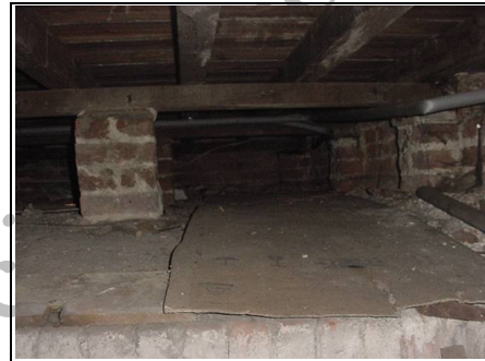
View under the floor
