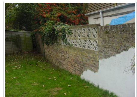
Rear boundary wall
