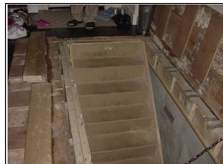
Stairs to basement
