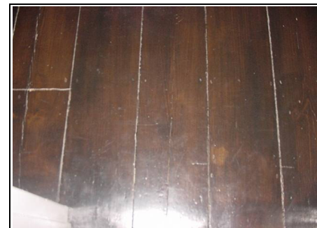
Floorboards to ground floor with light coming through
