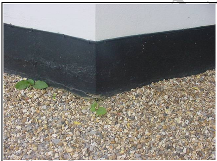
Base of property
