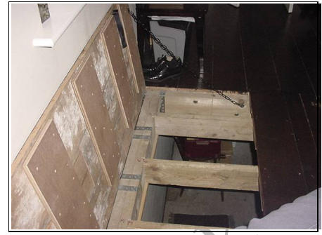
Ground floor being opened to reveal basement
