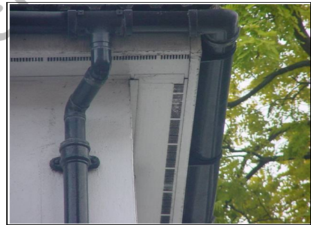
Fascias and Soffits
