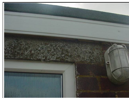
A close up view of the concrete lintel
