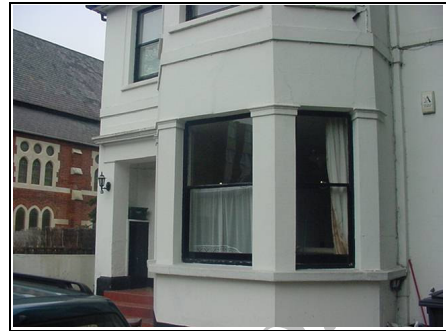
Timber sash window
