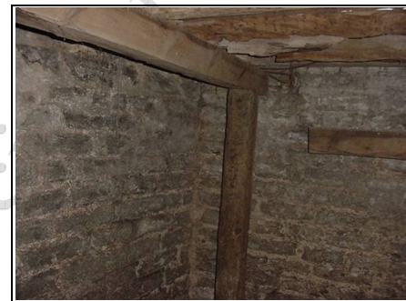
Long term additional support in cellar area to ground floor with dining room above
