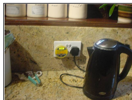
Earth test in kitchen
