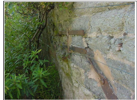
Bracing to wall
