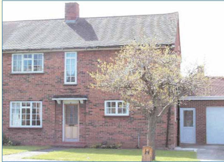
Bishops Drive Bishops Cleeve: metal framed casement windows 1948
