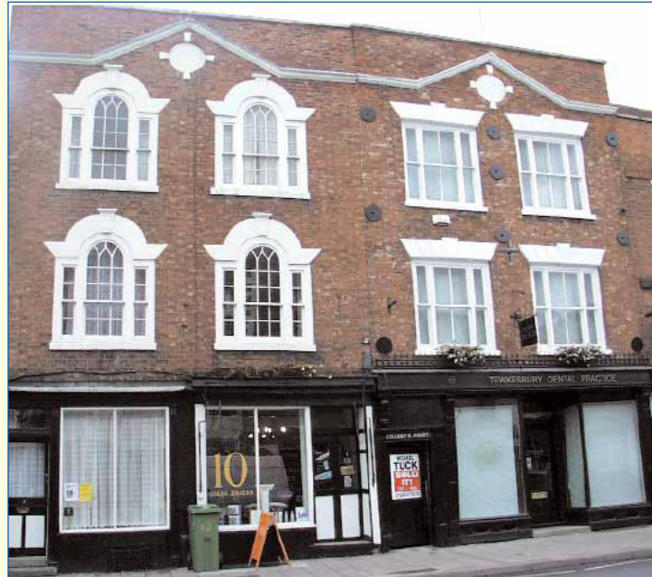
Late 18th Century curved gothic glazing bared sashes in 'Venetian' windows at 9 & 10 Barton Street, Tewkesbury with flush boxes. No 11 (right) has later 19th Century recessed tripartite sash windows
