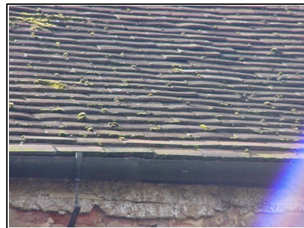
Old brickwork - was once render
