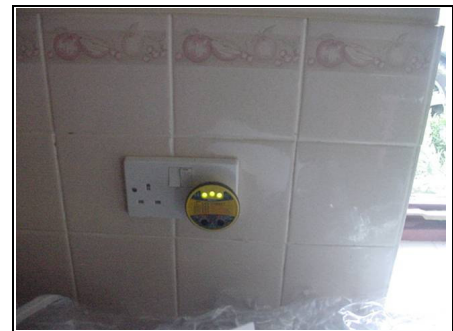
Earth test in kitchen
