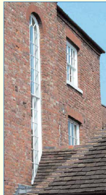
32 Church Street Tewkesbury: 1813 a remarkable elongated sash to light the staircase
