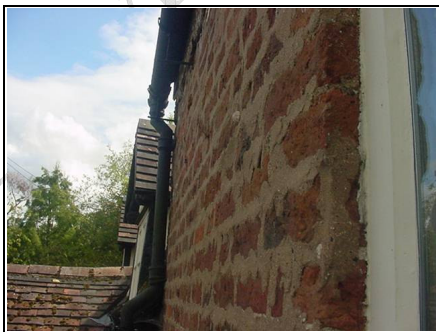
Old brickwork to rear
