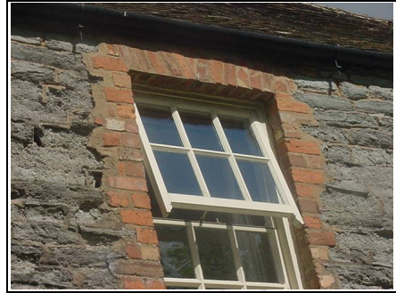
Double glazed windows - sliding sash look with a modern sash style
