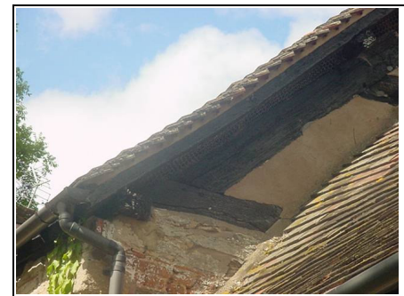
Upstand in roof
