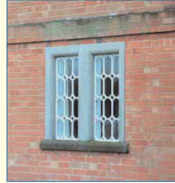
19th Century cast iron casements mimic leaded lights of previous centuries
