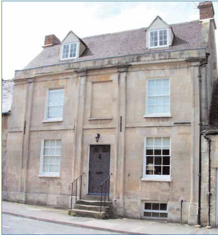
62 North Street Winchcombe: typical Georgian 6 over 6 sash windows
