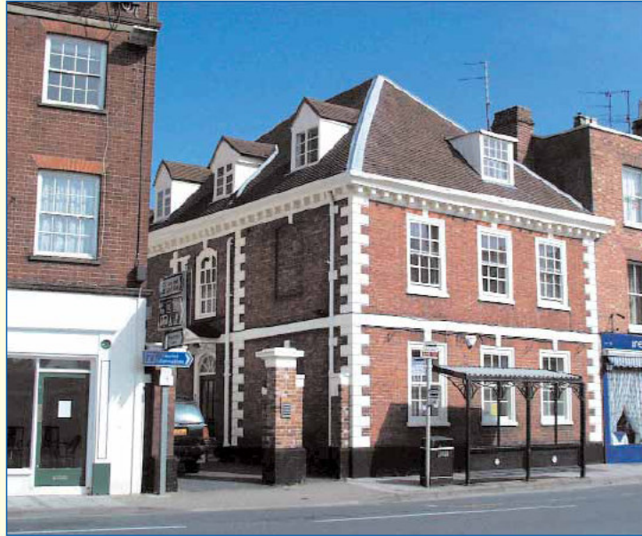
77 Church Street Tewkesbury: early 18th Century flush box sash windows
