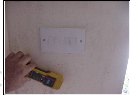
Checking for lateral dampness
