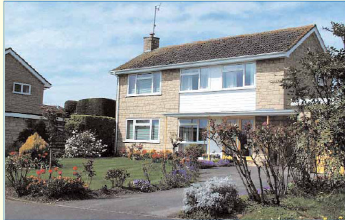
The Hyde Winchcombe: storm-proofed picture windows with top hung fanlights
