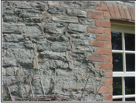
Deteriorating stonework
