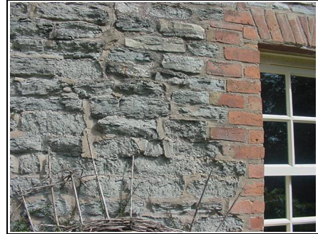
Deteriorating stonework
