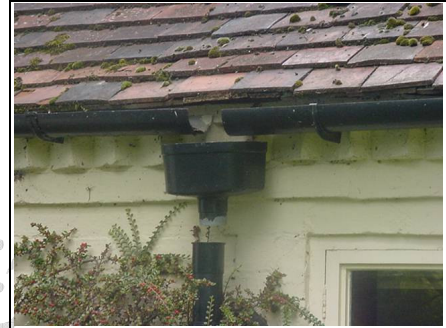
Gutters and downpipe and hopper head
