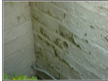
Brickwork around cloakroom
