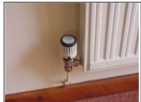
Earth test in kitchen
