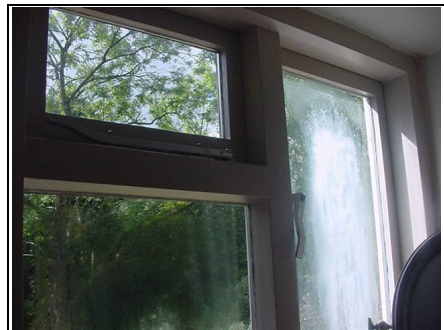
Misting up of double glazing
