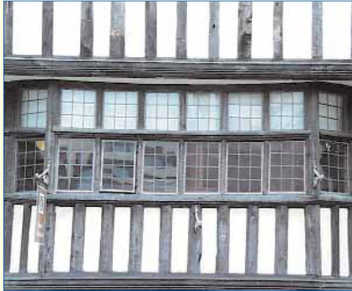
64 Barton Street, Tewkesbury: timber mullioned & transomed windows 17th Century
