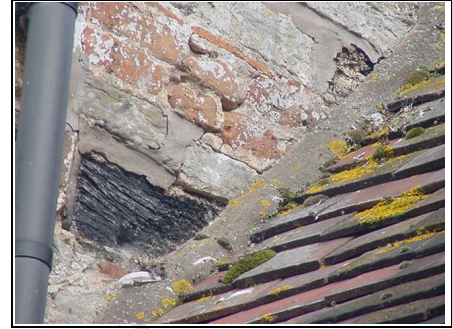
Cement flashing
