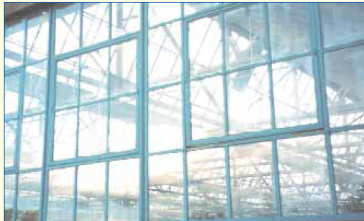
Crittall windows: GAC Gloucester Aircraft Co. Brockworth
