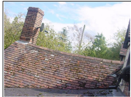
Roof over cloakroom
