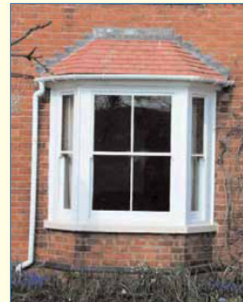
Ropewalk Tewkesbury: Victorian sash with horns
