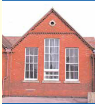
1905 Chance Street Primary School Tewkesbury: concealed box sash windows with horns
