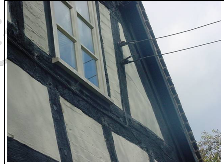
Timber fascias and soffits
