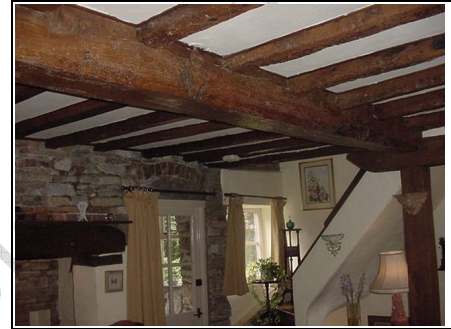
Spine beam with exposed floor timbers
