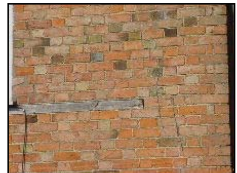
Flemish Bond brickwork to the gable end and also the bonding timbers.
