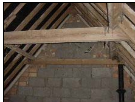
The party wall, which is block work.
