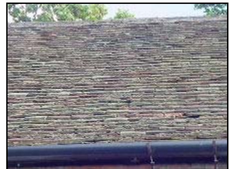
A general view of the roof.
