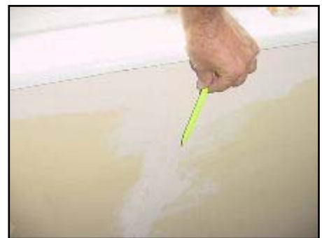
Internal cracking
