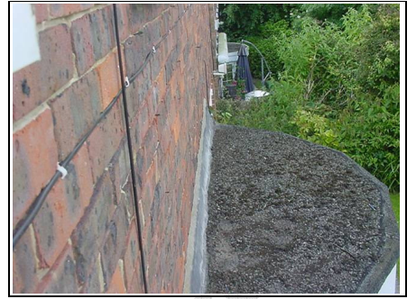
Bow window roof
