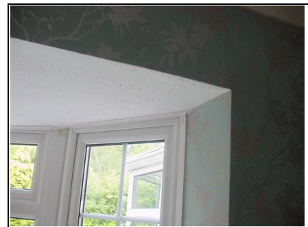
Looking for lateral dampness underneath bow window – no visible signs
