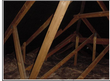
General view of inside of main roof
