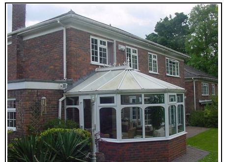
Kitchen/Conservatory to the rear
