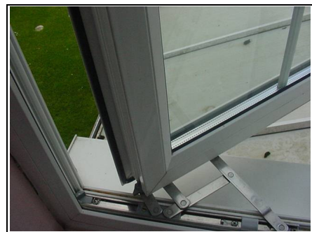
Close up of double glazing
