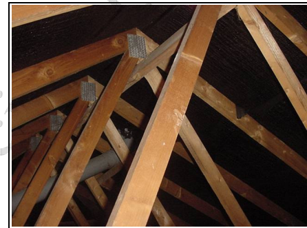
Pre-fabricated truss roof
