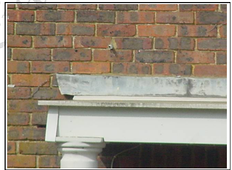
Roof over entrance porch
