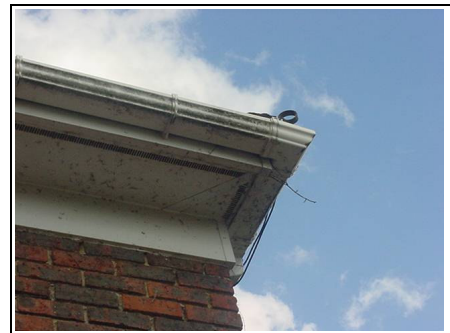
Close up of Gutter
