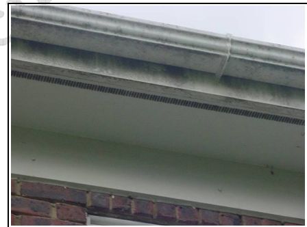
Fascias and soffits
