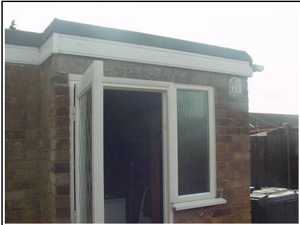
A rear door to a 1970's building. Can you tell where the cold bridging would be in this photo?
