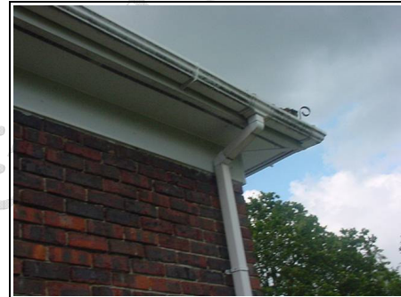
Gutter and downpipe
