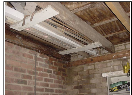
Rear right hand corner of garage roof
