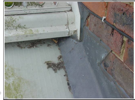
Close up of lead flashing where conservatory meets the main building
