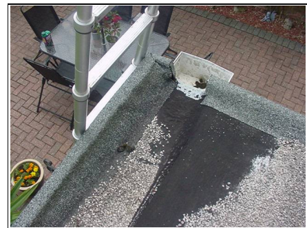
Right hand side flat roof 15
