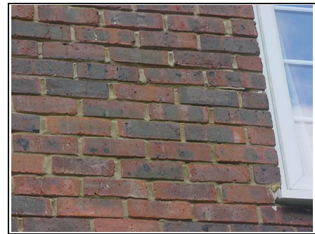
Brickwork with poor quality pointing
