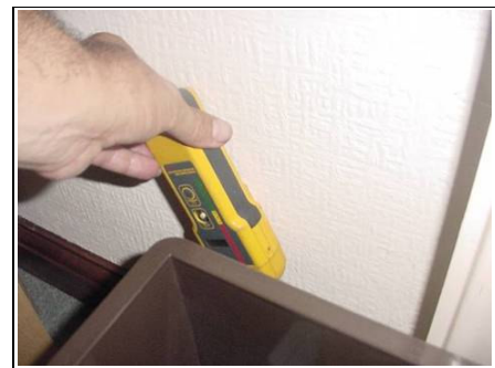
Checking for rising damp
