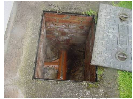
Manhole to rear middle of property
