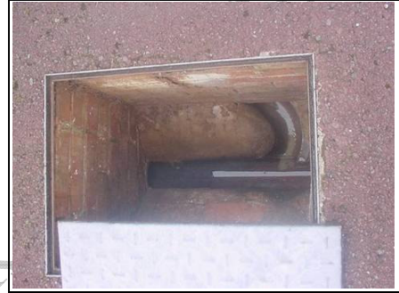
Manhole to rear
