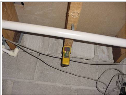
Checking timbers in ceiling void
