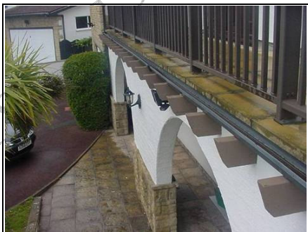
Concrete rafter feet on balcony
