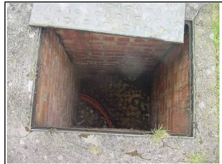
Manhole to rear left hand corner
