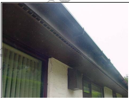
Plastic profile guttering
