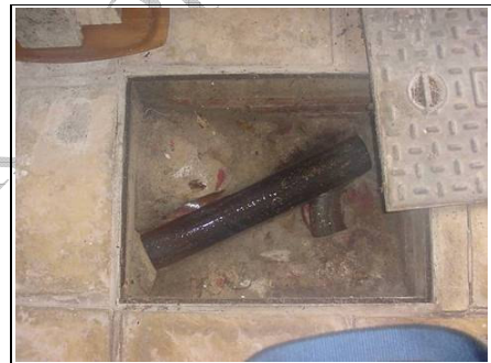
Manhole to front, near study
