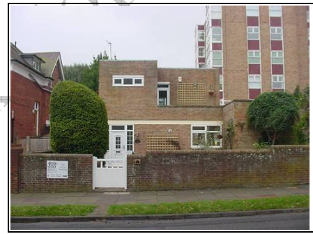
1960's concrete frame
