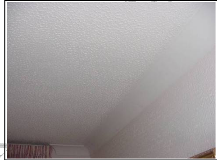
Textured ceiling finish
