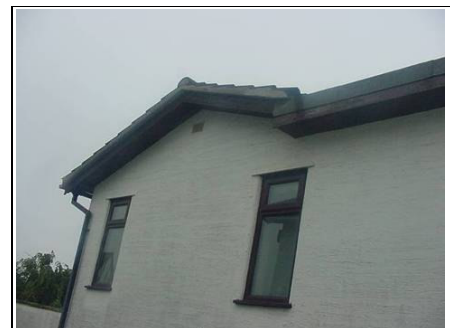
Two plastic double glazed windows to front of property
