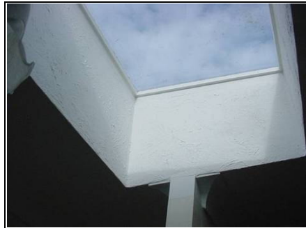
High Level Roof Window above Shower Room
