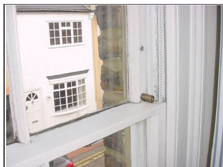
Sliding sash window to front
