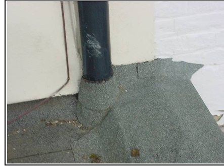
Felt flashing meeting main property
