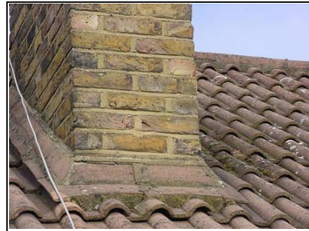
Base of chimney with a tile on edge flashing
