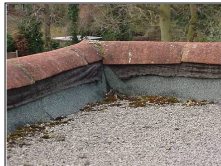
Flashing deteriorating
