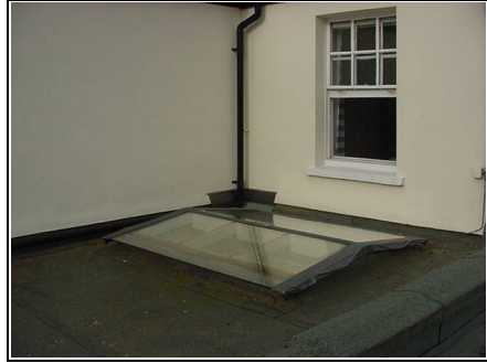
Low level flat roof
