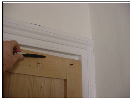
New doors fitted into old frame
