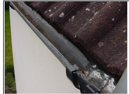
Gutter – repaired with Flashband
