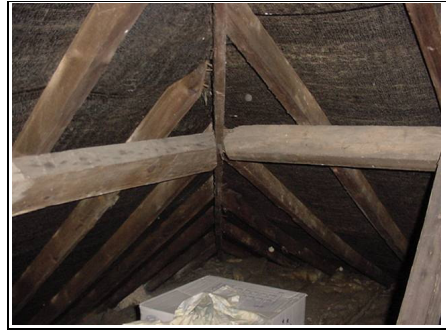
General view of the hip, showing some movement – we would term this as old and established.
