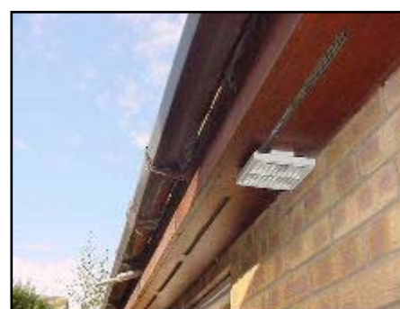
Vented soffit to the left hand side.
