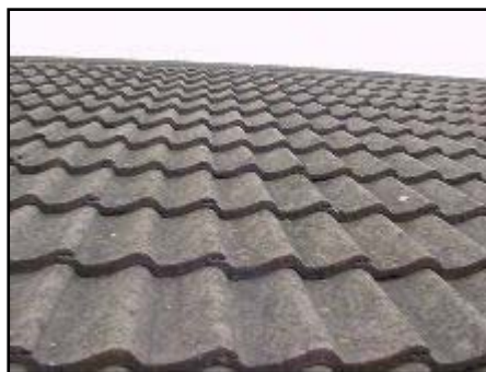
This is a close up view of the roof.
