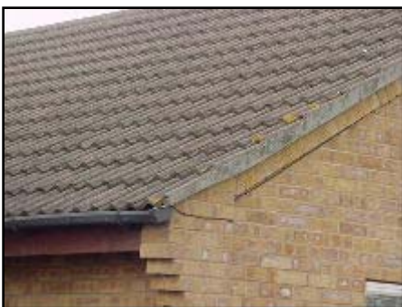
A general view of the roof.
