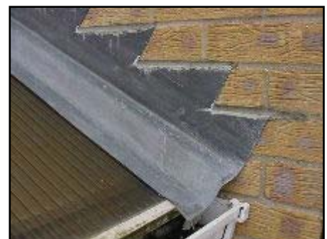
Close up of lead flashing.
