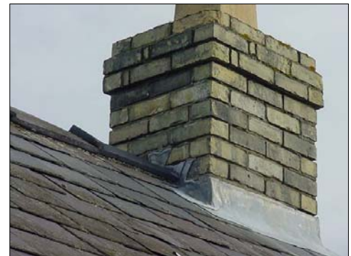
Rear view of the chimney.
