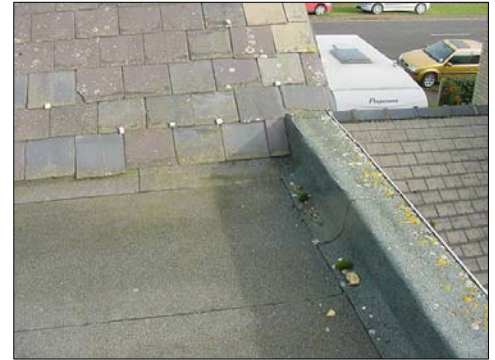
A view of the high level parapet wall.
