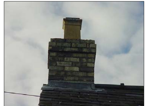
Front view of the chimney.
