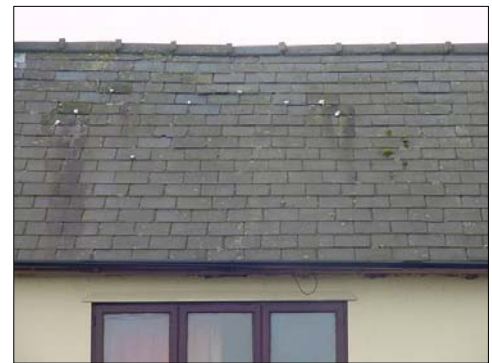
A view of the main roof with some lead tingles.
