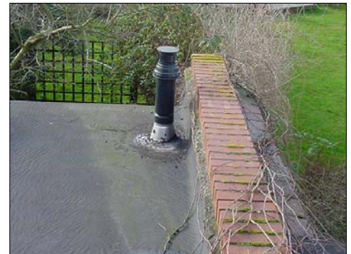
A general view of the parapet wall.
