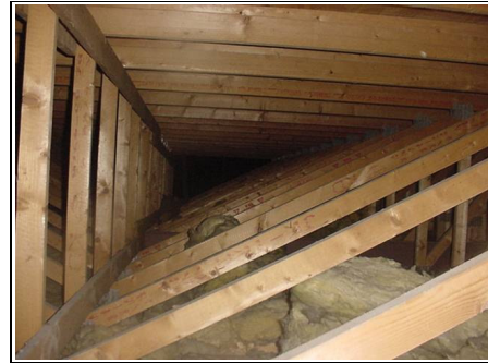
Inside main pitched roof
