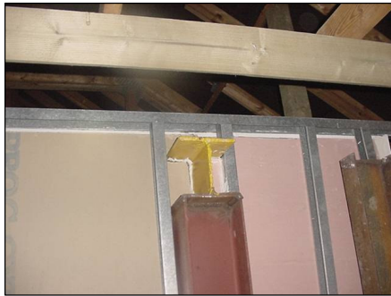
Photograph shows steel structure
