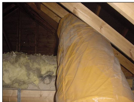
Roll of insulation waiting to be laid in roof
