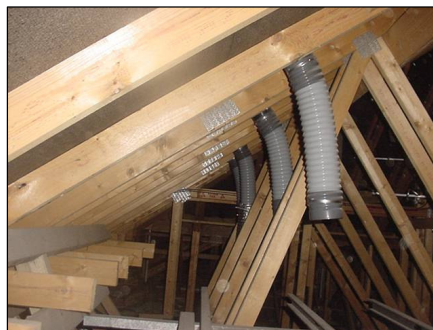
Tubes within roof
