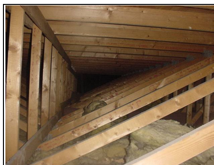
Inside main roof
