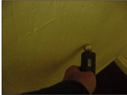
Checking for lateral dampness in basement
