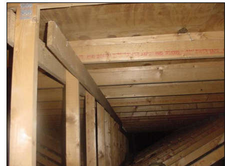
Inside flat roof
