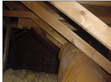
Insulation still in a bag ready to be laid!
