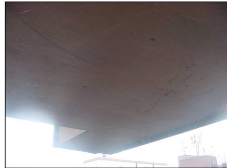
Soffit taken through the window on the lift landing
