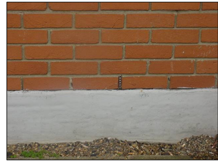
Close up of brickwork
