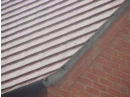
Cement verge with smaller tiles
