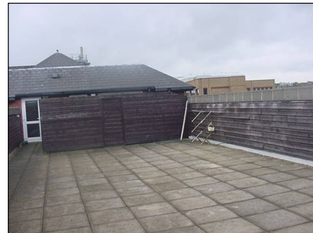
Flat roof area
