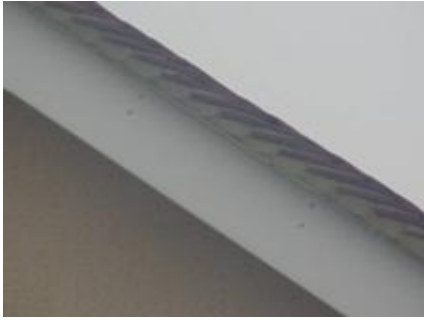
Cement verge with smaller tiles
