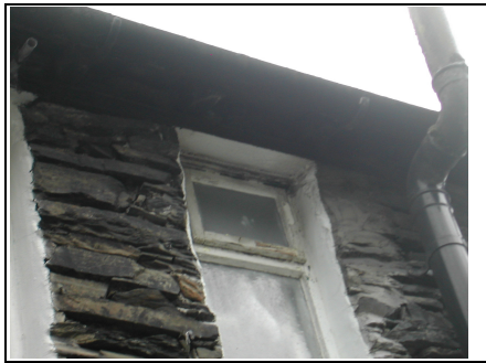
Windows in poor condition
