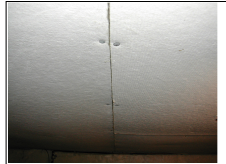
Ground floor concealed by boarding in the cellar
