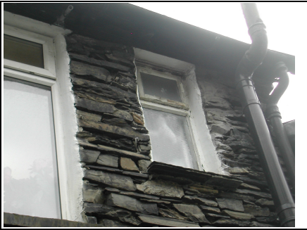
Plastic soil and vent pipes
