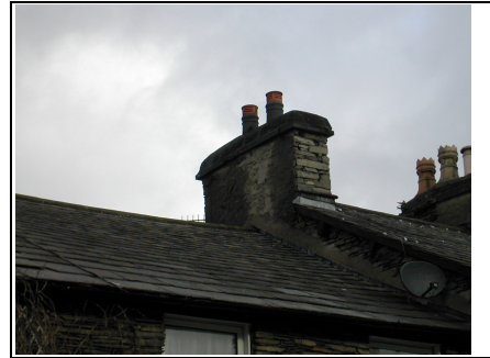
Front view of chimney
