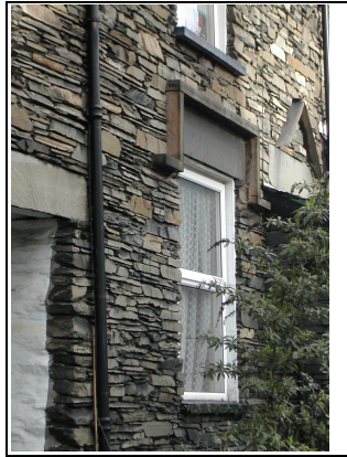
Front elevation wall with large lintel above
