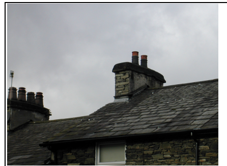
Front view of chimney
