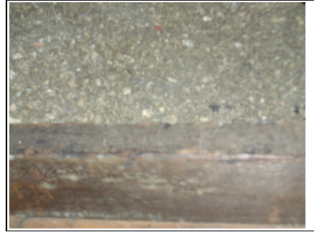
Joist and loose fill insulation
