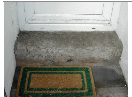
Crazing to front door step
