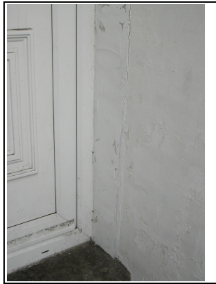
Hairline cracking around door frame
