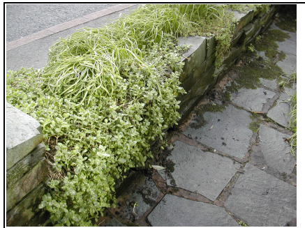
Stone wall covered in vegetation
