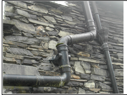
Plastic soil and vent pipes
