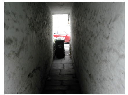
Passageway to rear
