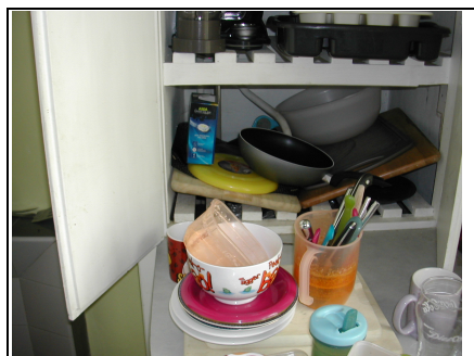
Hot water cylinder is in kitchen cupboard
