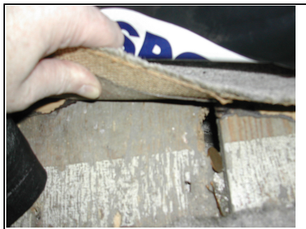
Signs of woodworm activity in front bedroom floor
