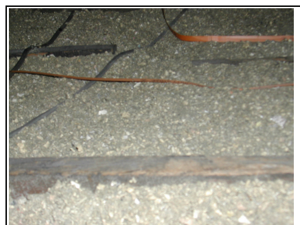
Loose fill roof insulation
