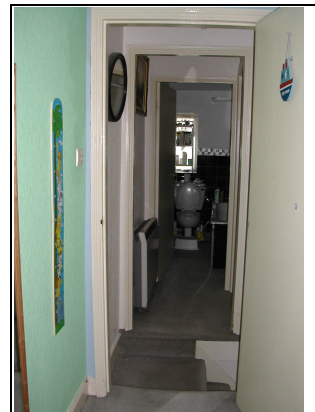
First floor wall above chimney breast
