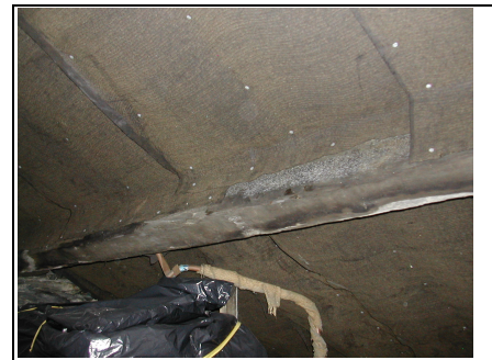
Rear roof pitch
