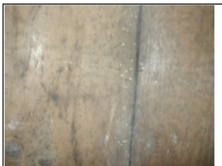
Signs of woodworm activity in the floor
