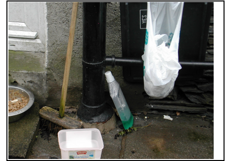
Combined drainage entering the ground
