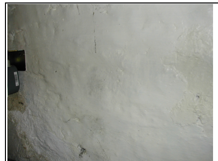
Wall in cellar beneath chimney breast above
