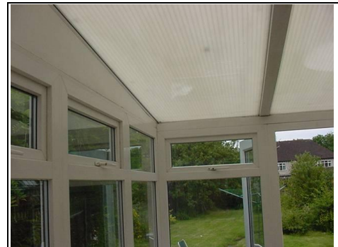
Polycarbonate roof
