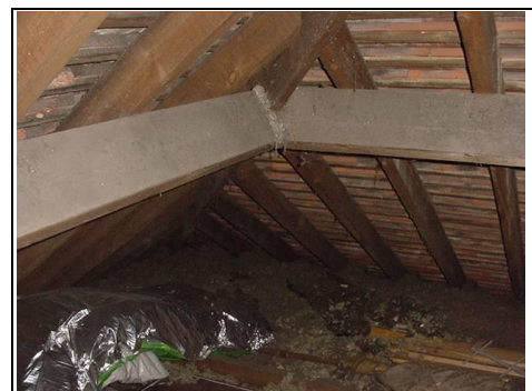
Hip of the roof
