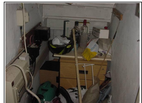
The stairs are not lined
