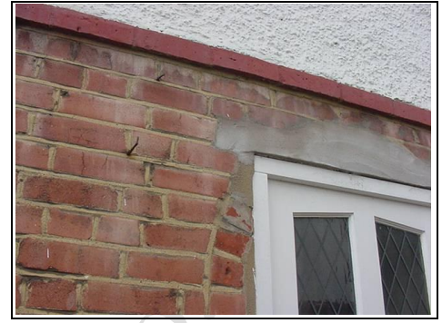
Lintel altered to the left hand side
