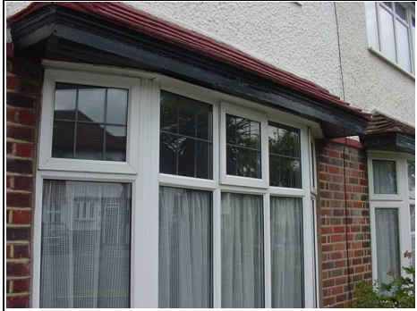
Bay window roof
