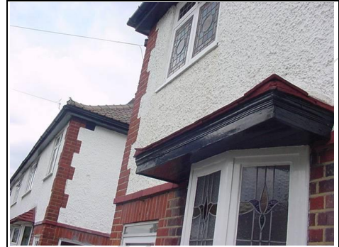
Bay window roof
