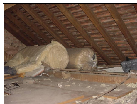
General view of the roof
