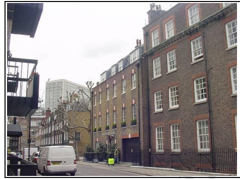
Older style London converted flats with property problems such as Condensation and Cold Bridging
