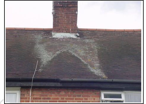
There is a dip in the rear roof
