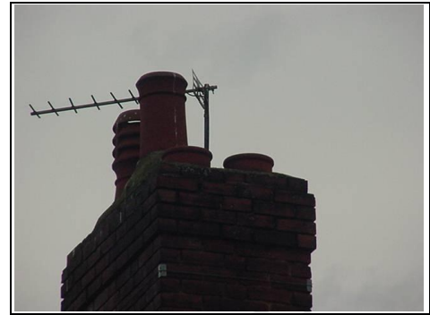
Top of right chimney
