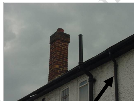
Gutter and downpipe
