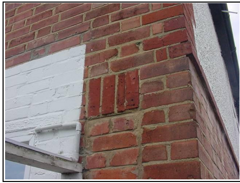
Lintel altered to the rear
