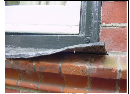
Lead window sill
