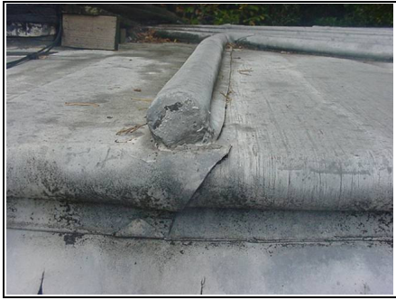
Lead work –roll joint
