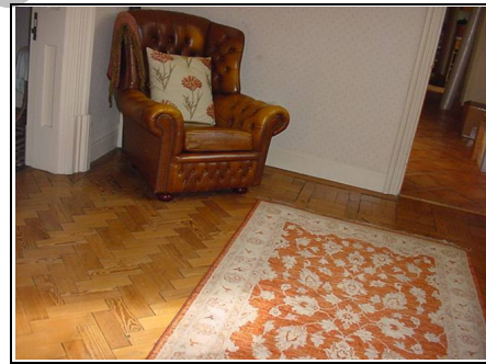
Wood block flooring over suspended timber floor
