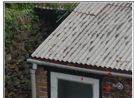
Asbestos roof on garage
