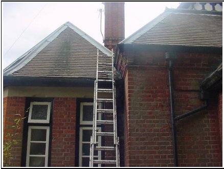
Access to valley gutter
