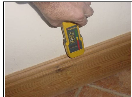
Testing for rising damp
