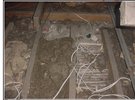
Lath and plaster ceiling
