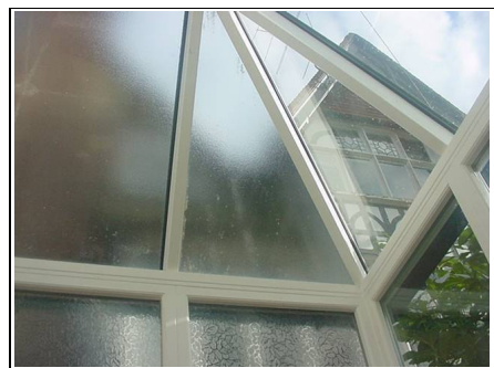
Opaque glass to left hand side and clear glass to right hand side
