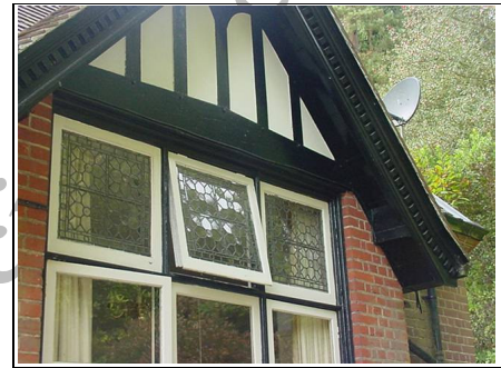
Fascias and soffits painted black
