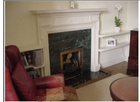
Fire in lounge partly closed
