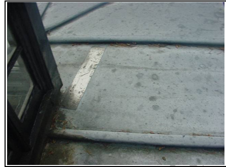
Lead roof with temporary sticking plaster Flashband repair
