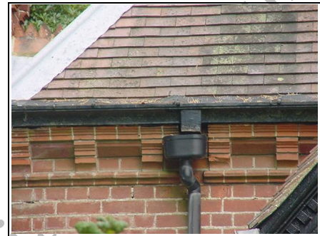
Metal gutter and plastic downpipe
