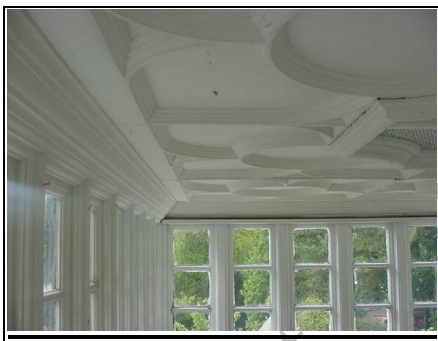
Moulded plaster ceiling
