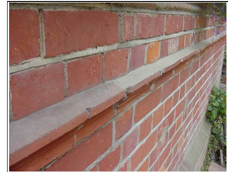
Repair to rubbed brick
