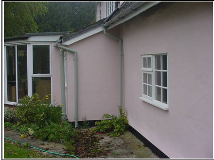
Downpipes discharging to rear left hand side
