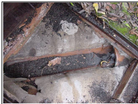
Drain one to rear right hand side
