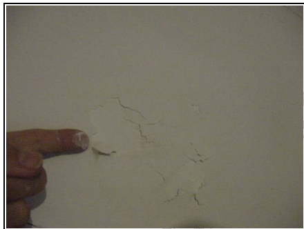
Old lime wash within utilities room
