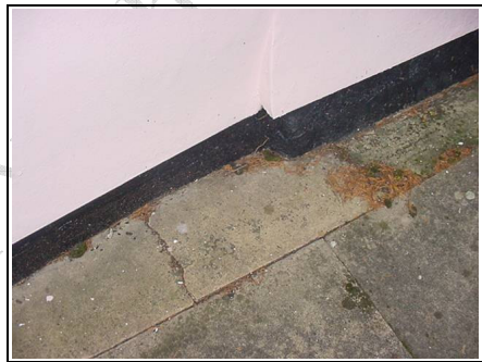
Concrete surrounding building
