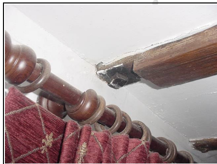
Metal ties / restraints visible to floor joists
