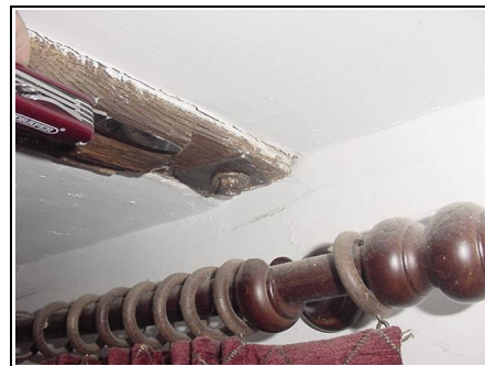
Metal ties / restraints visible to floor joists
