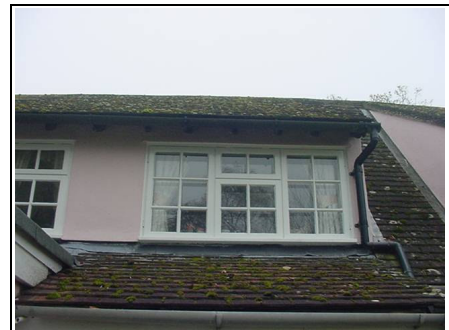
Rear dormer windows
