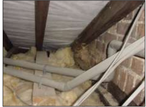
Close up of common rafters checking rear detail
