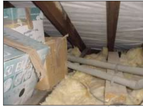
Inside the roof
