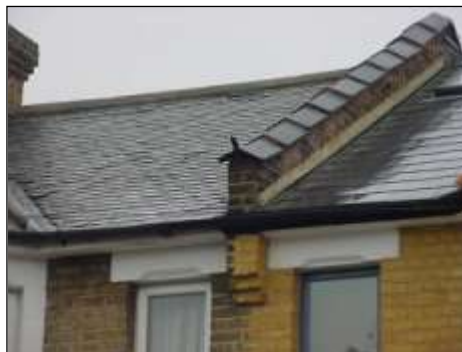
Parapet wall left hand side
