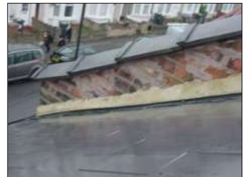
Parapet wall close up your side
