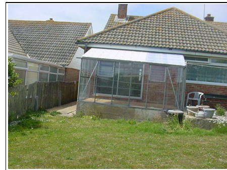
Greenhouse with concrete raft foundation
