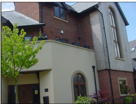
Timber cladding brickwork and render mixed
