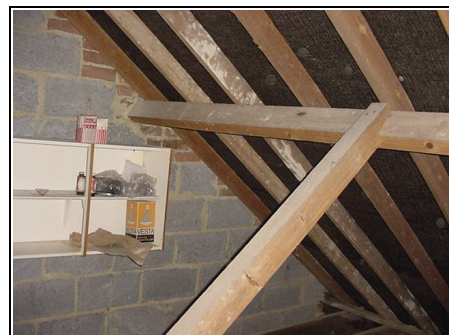
Roof general view with a new prop (diagonal timber)
