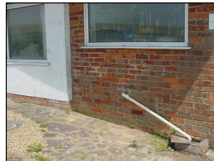
Airbrick also showing slope of the ground
