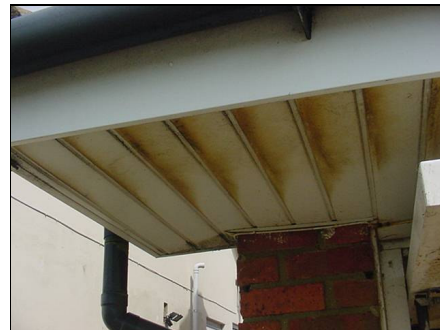
Close up of cladding
