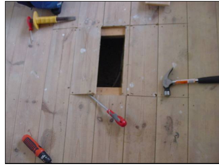
Lifting up floor in the left hand side bedroom
