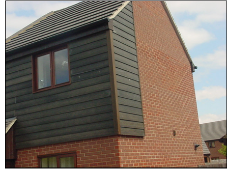
Plastic cladding dark timber coloured
