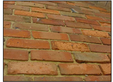
Close up of brickwork
