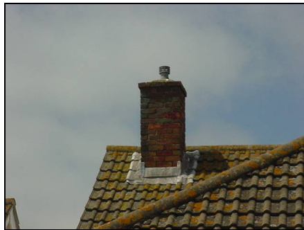
Chimney One right hand side chimney one viewed from the rear
