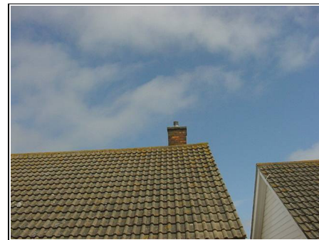
Concrete roof tiles
