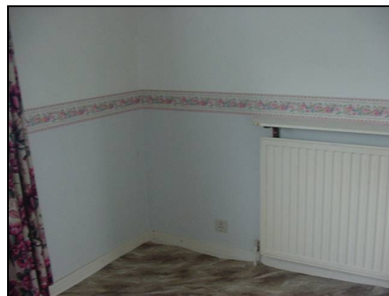
Internal single panelled radiator
