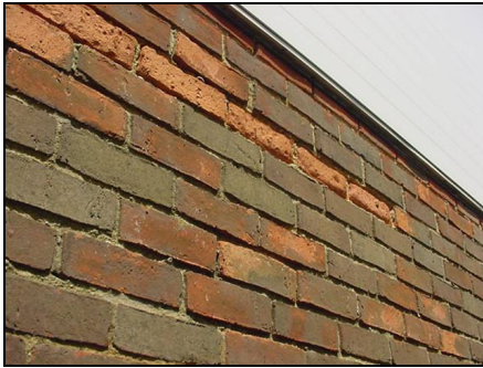
Brickwork right hand side
