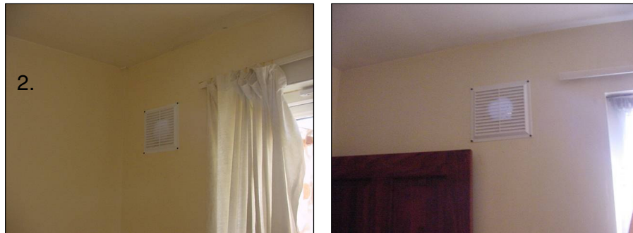
Vents within bedroom
