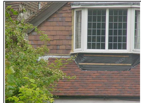
Work required to window
