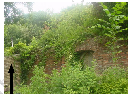
Shed to left hand side
