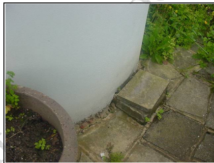
Front right hand side semi-circular bay
