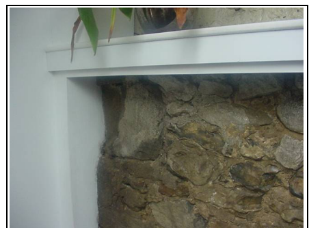
Exposed stonework in Shower room
