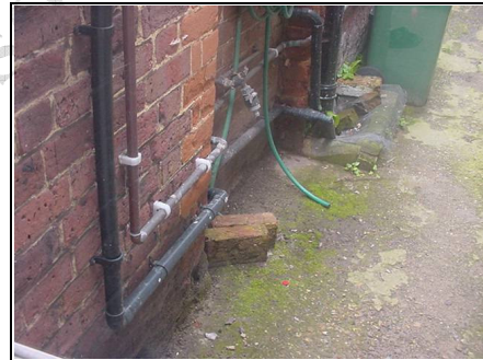
Soft red brick with moss sitting against it. Moss indicates not much sunlight gets in. Ground needs lowering
