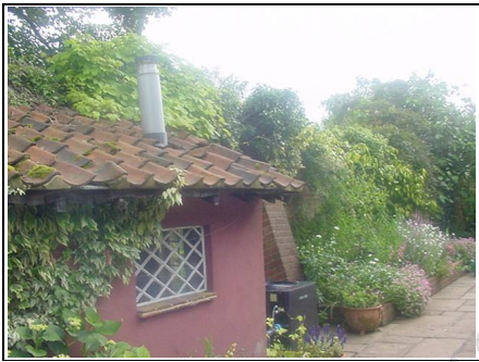
Swimming pool outbuilding which has been in place for 30 years
