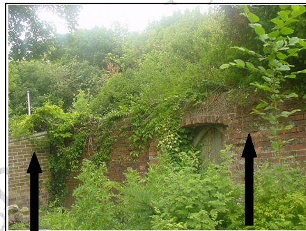
Shed to left hand side, repointing required to right hand side of gate
