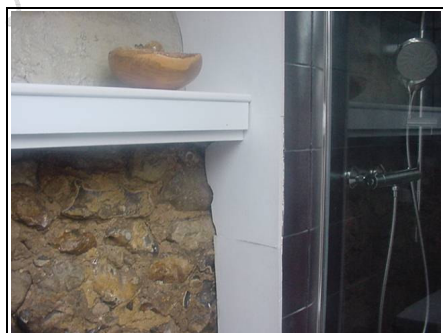
Exposed stonework in Shower room
