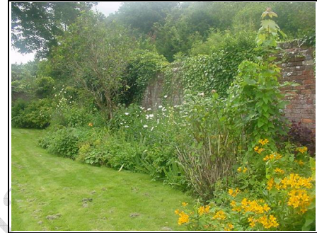
Right hand boundary wall
