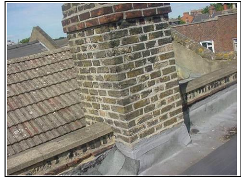
The chimney has felt flashing around it
