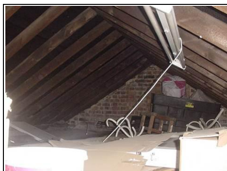
General view of the roof
