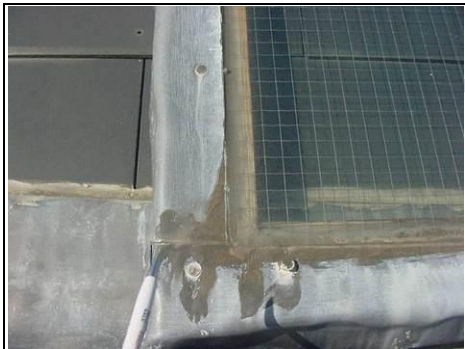
Mastic sealing to access area
