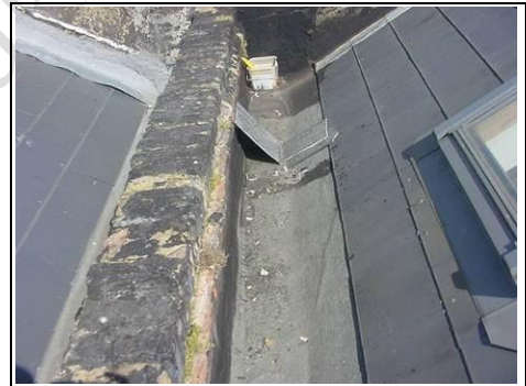
Bitumen paint used
