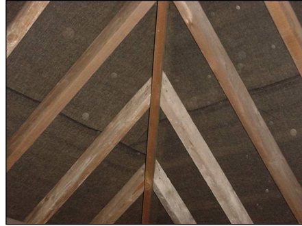
Looking at the rear left hand hip of the roof
