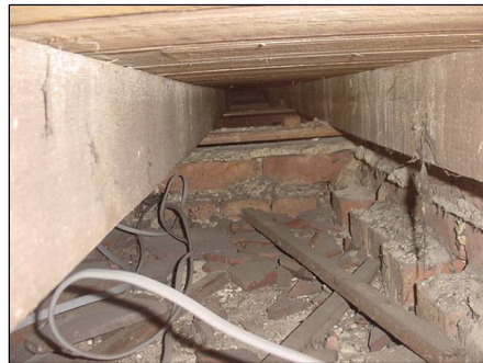
Suspended timber floor sitting on to the sleeper wall
