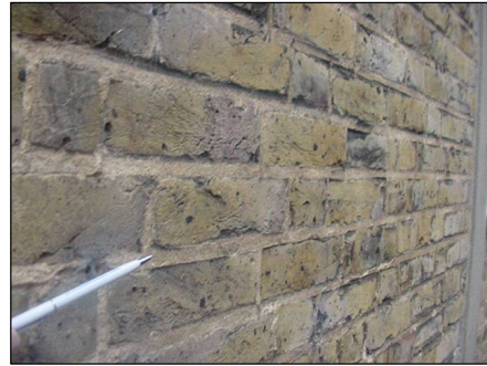
Cement pointing to brickwork
