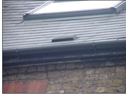
Low level vent only visible to the loft conversion
